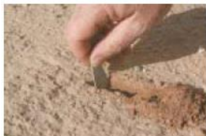
Figure 1. Excavate small trench.
