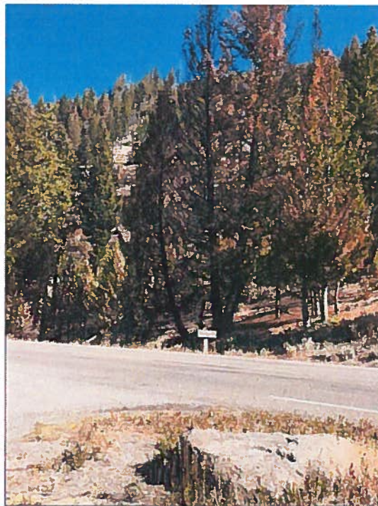
Figure 17. Maple fire disturbance along roadside where hazard tree mitigation is needed.
