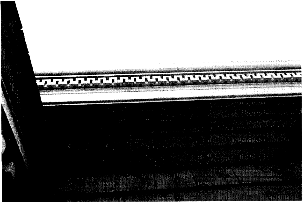
Illustration 39. Penniman House: Trim at Curb of Mansard Roof (1984).
