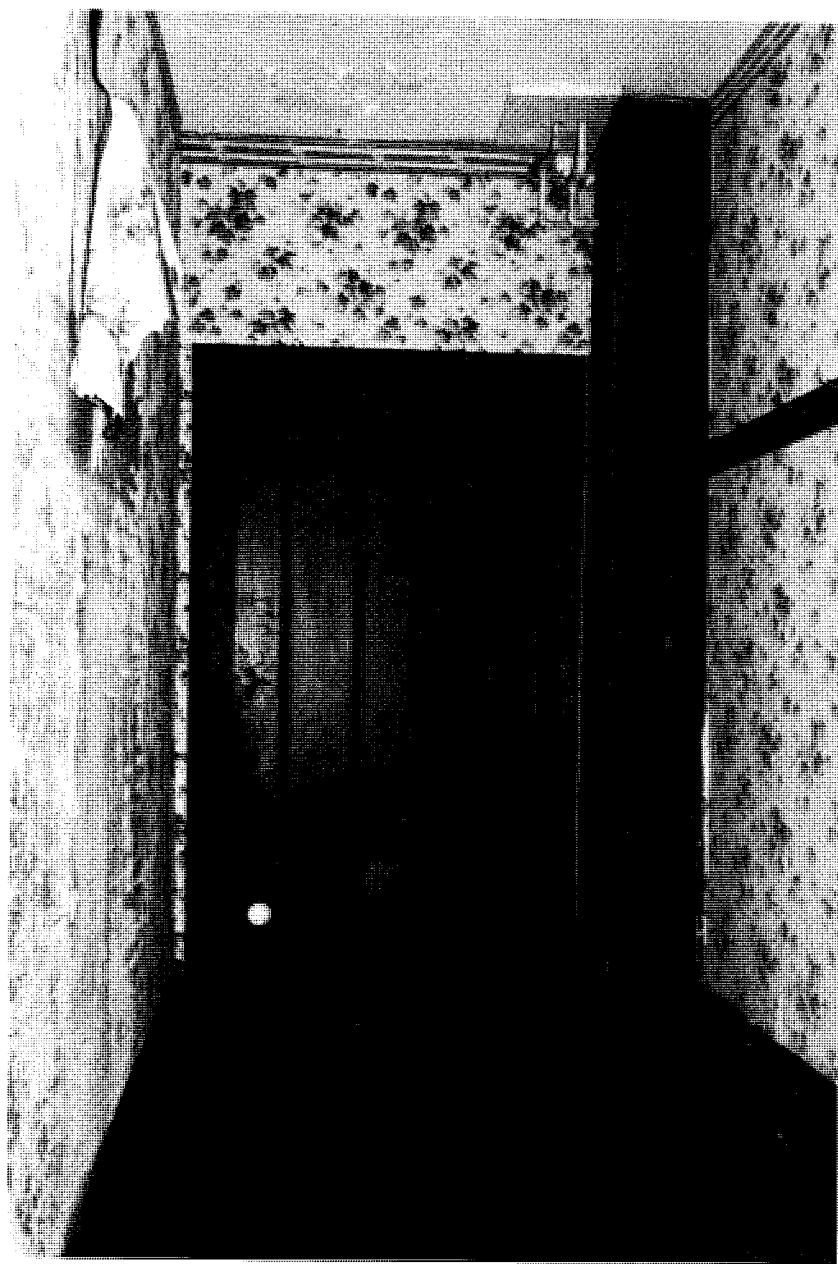
Illustration 99. Penniman House: Back Hall (Room 105), North Wall, Showing Pipe Chase (1984).
