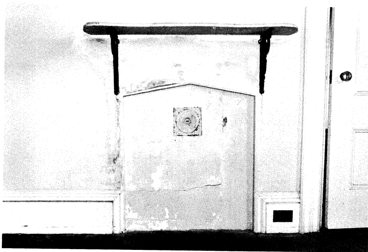
Illustration 67. Penniman House: Southwest Parlor (Room 101), East-Wall Mantelshelf, Stovepipe Thimble, and Cover (1984).
