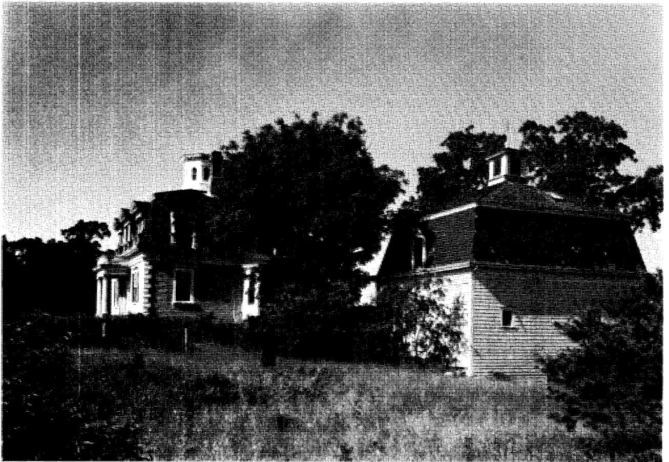
Illustration 26. Penniman House: West and South Facades of House and Barn (1962).
