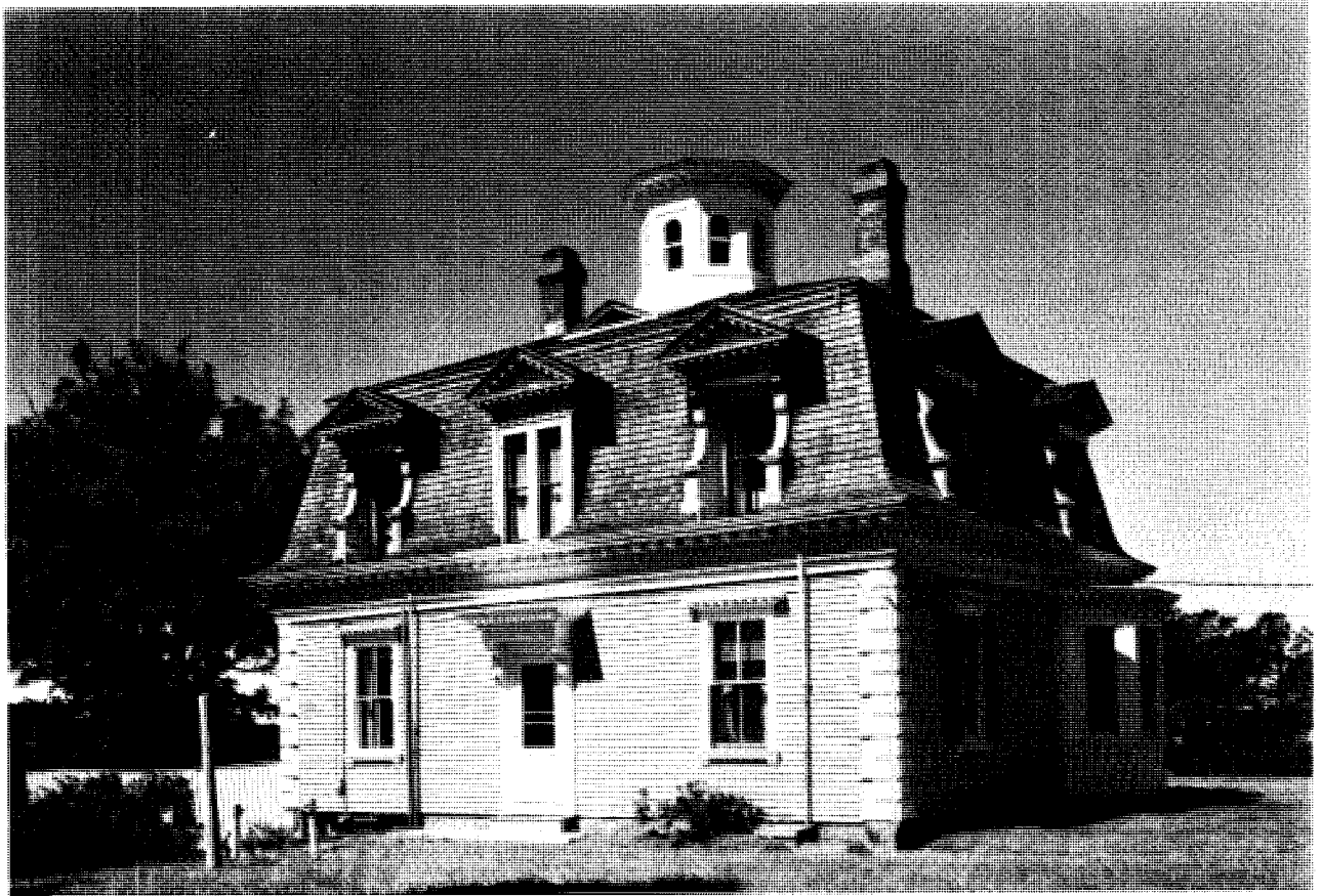
Illustration 23. Penniman House: East Facade (1962).
