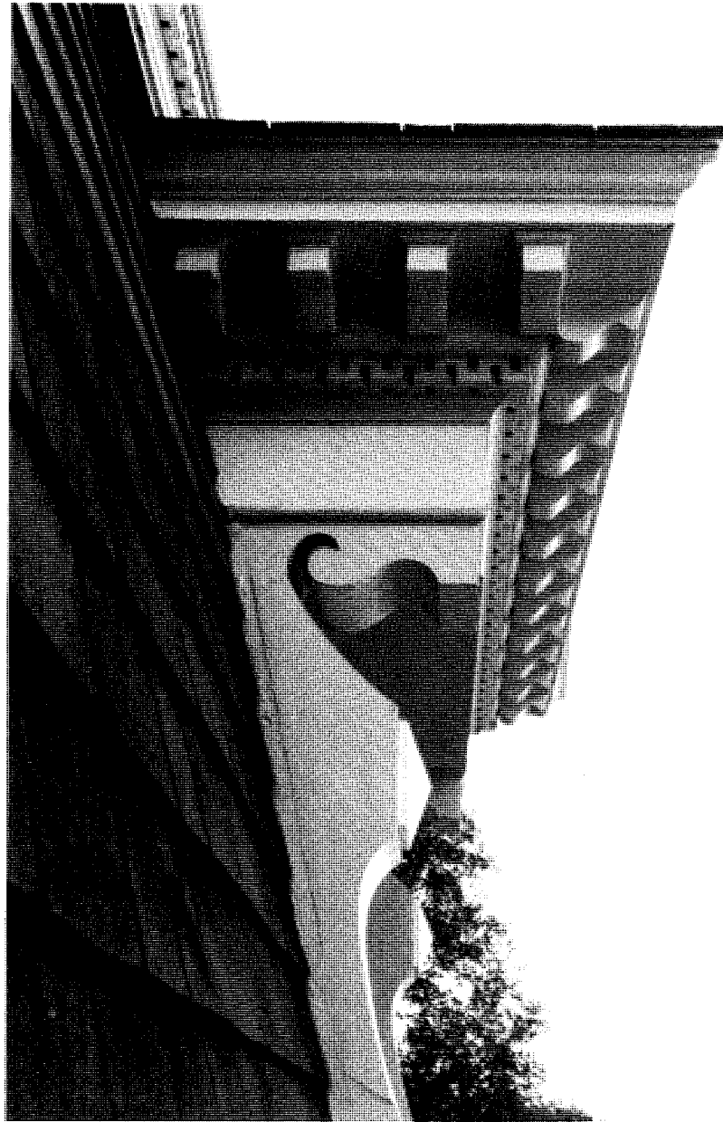
Illustration 27. Penniman House: Detail of Typical Dormer-Window Hood (1984).
