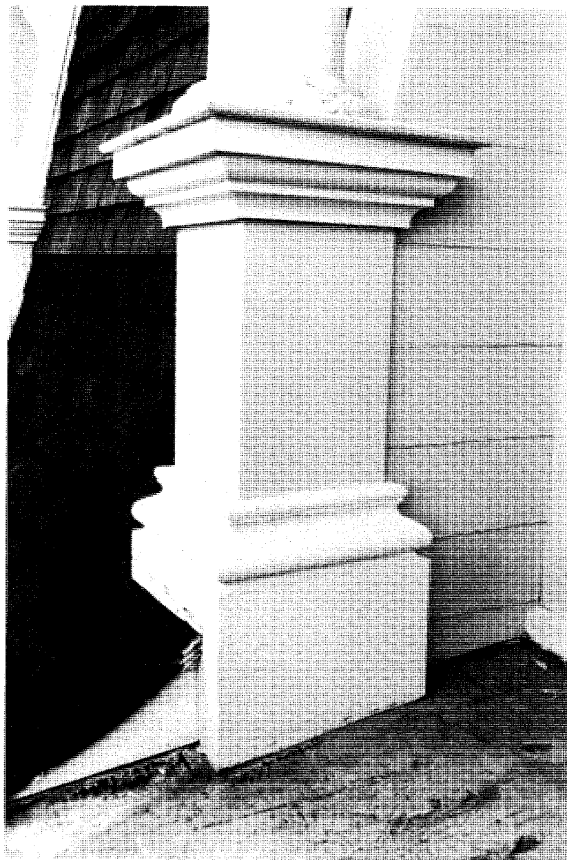
Illustration 29. Penniman House: West Facade, Pedestal for Colonette of Center Dormer Window (1984).
