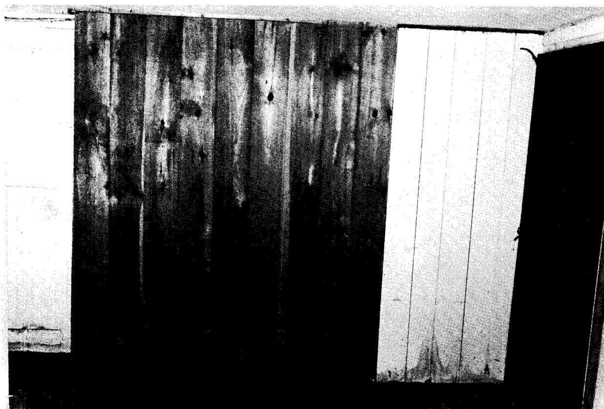
Illustration 54. Penniman House: Finished Basement Space (Room 001), Looking East at Partition Forming Room 002 (1984).
