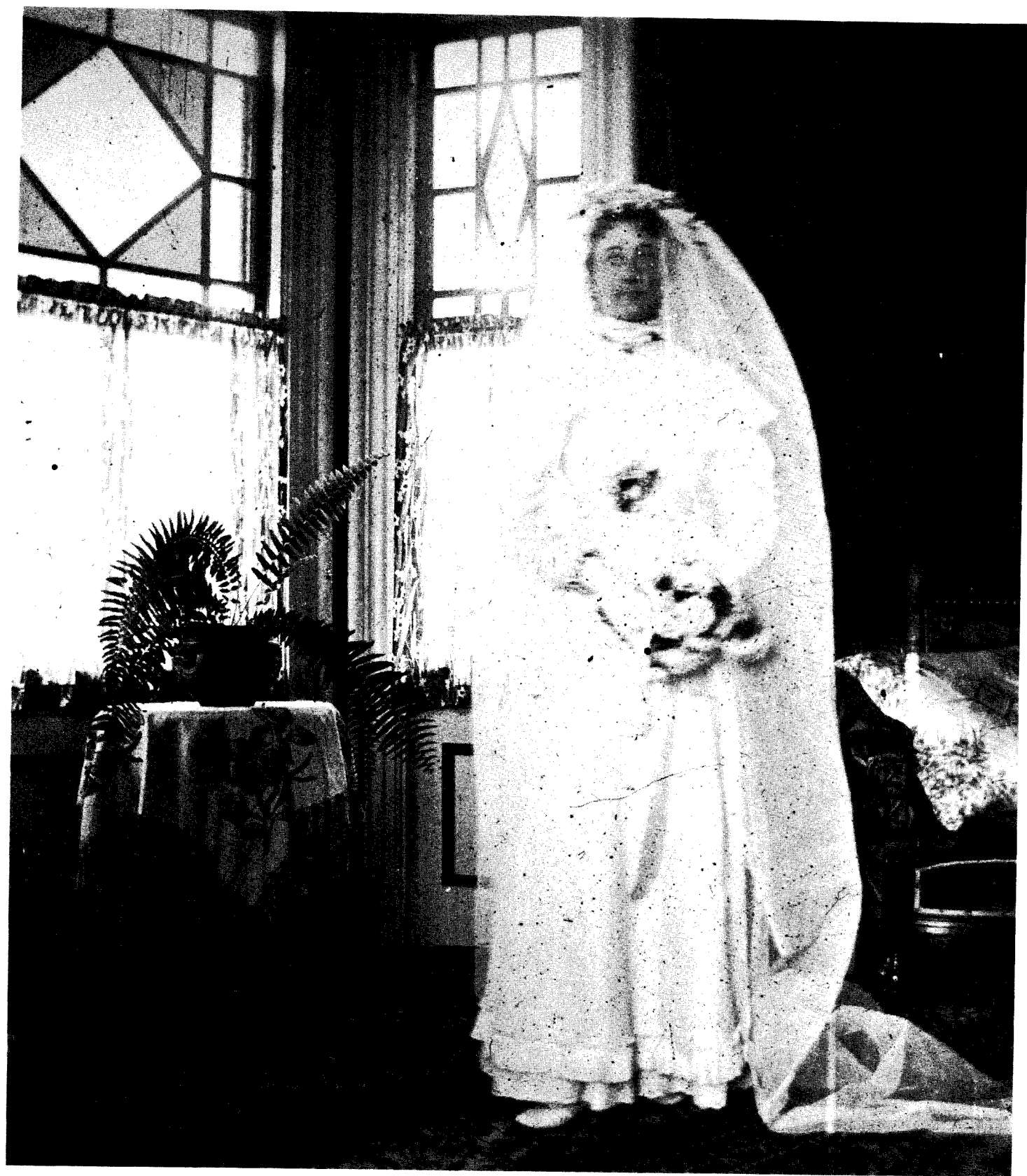
Illustration 76. Penniman House: Northwest Parlor (Room 103), North-Wall Bay Window (Circa 1890).
