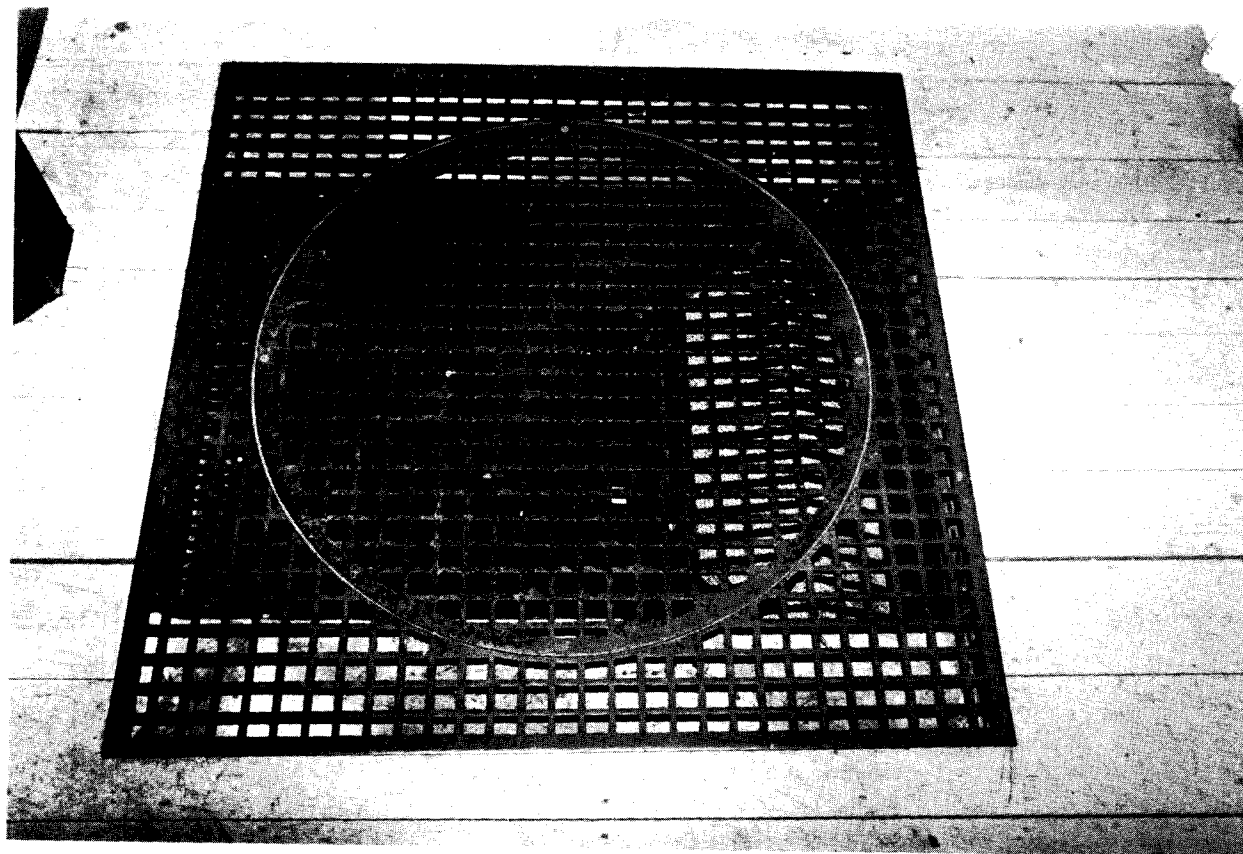
Illustration 72. Penniman House: Front Hall (Room 102), Circa-1940 Hot-Air Floor Register (1984).
