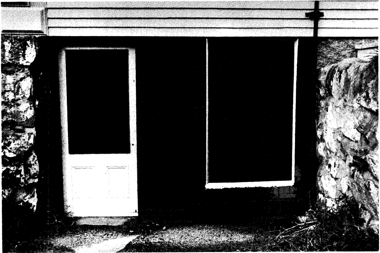
Illustration 14. Penniman House: East Foundation Wall, Showing Basement Doorway and Window (1984).
