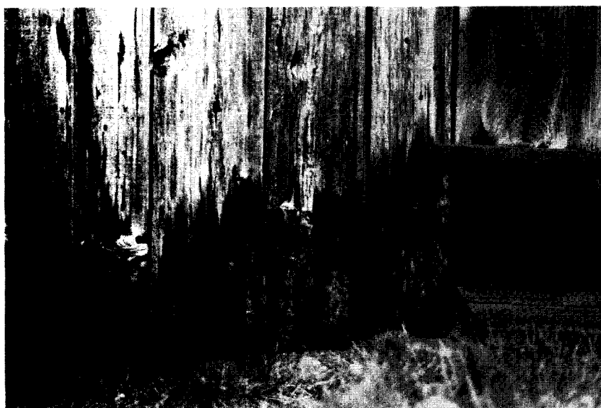
Illustration 104. Atwood-Higgins Barn: Rising Damp and Fungal Growth.
