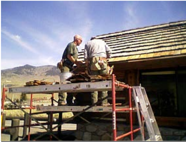
Red Williams & Mike Laye repairing the North Entrance roof Wednesday. Photo by Tonya Mathews.
