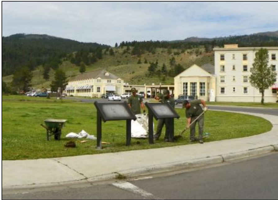
Boardwalk crew installing new wayside exhibits at Mammoth to interpret elk natural history and visitor safety. The exhibit was designed by exhibit staff and reviewed by subject matter experts. (photo by Jo Suderman)
