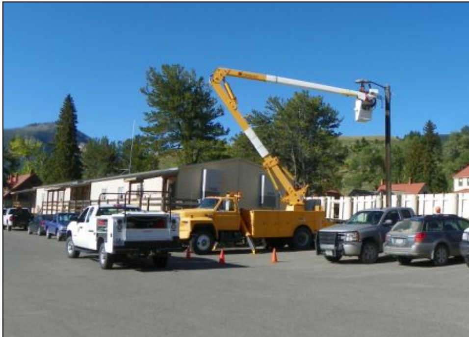
Shawn Morrison replacing an existing light fixture with a directed light fixture (photo by Jo Suderman)
