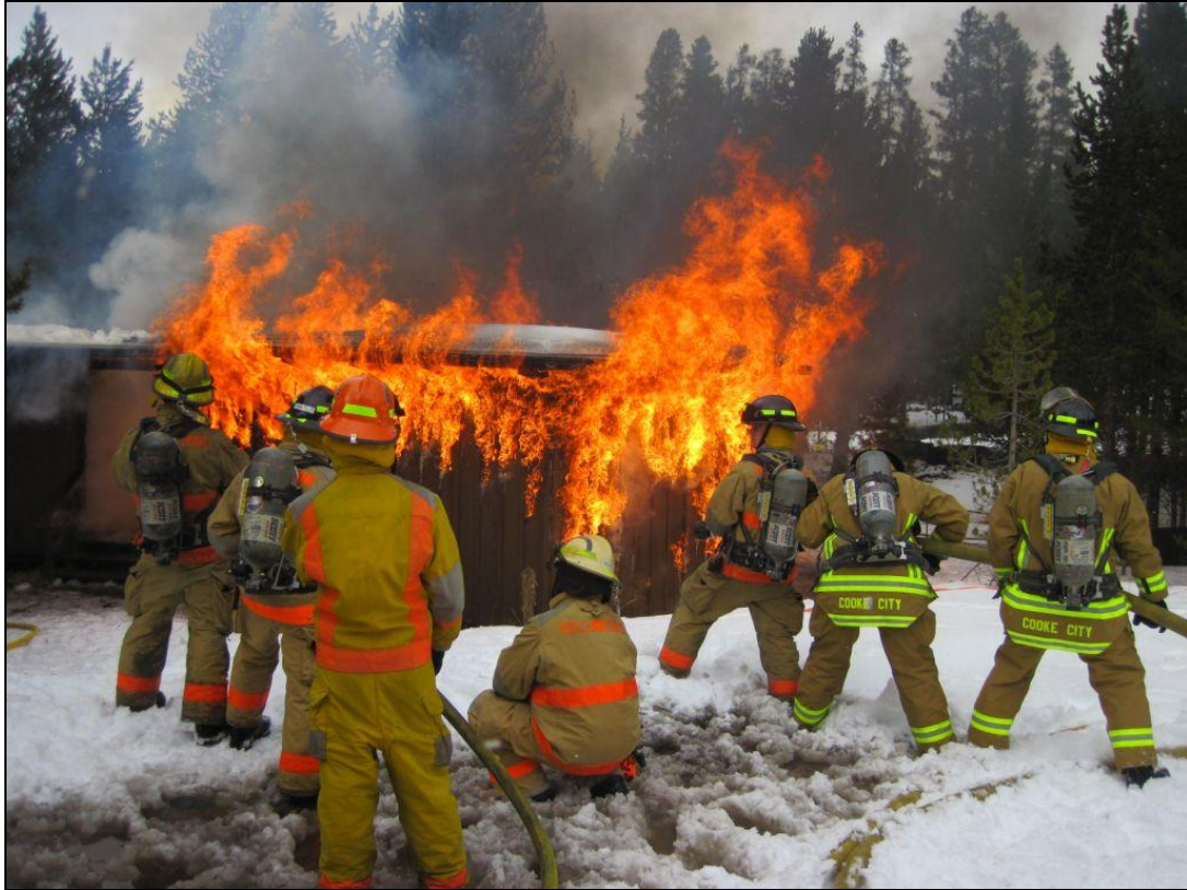
The Yellowstone and Cooke City Fire Companies were able to perform some live fire training this weekend at the Canyon cabin area thanks to some planned cabin demolition. (photo by Jerry Bartlett)
