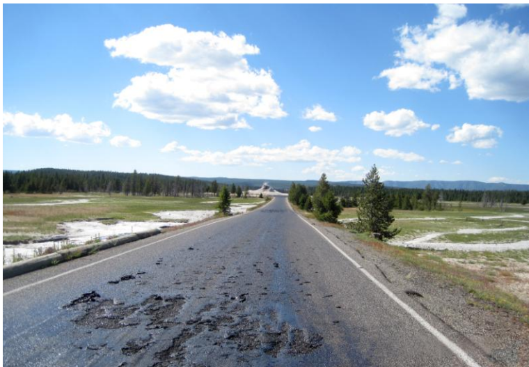
Firehole Lake Drive, superheated by surrounding thermals. (NPS Photo)
