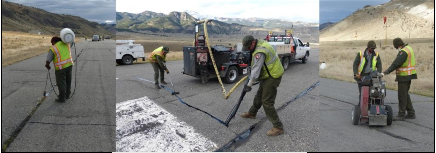
NPS crew crack sealing the Gardiner Airport runway. (photo by Al Nash)
