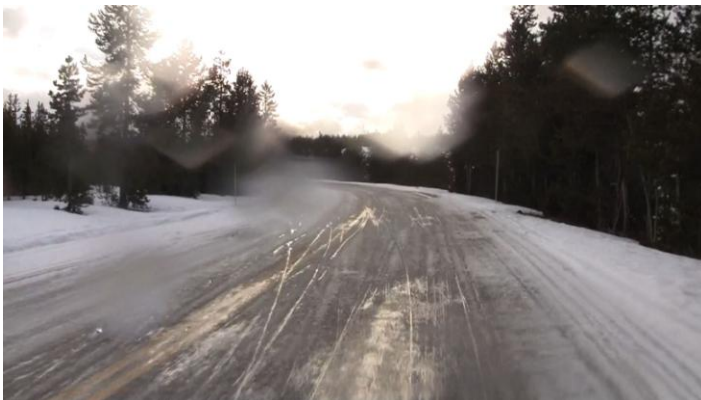
The road centerline and sections of wet pavement are clearly visible in this image taken along a section of the road linking West Yellowstone and Madison Junction.
