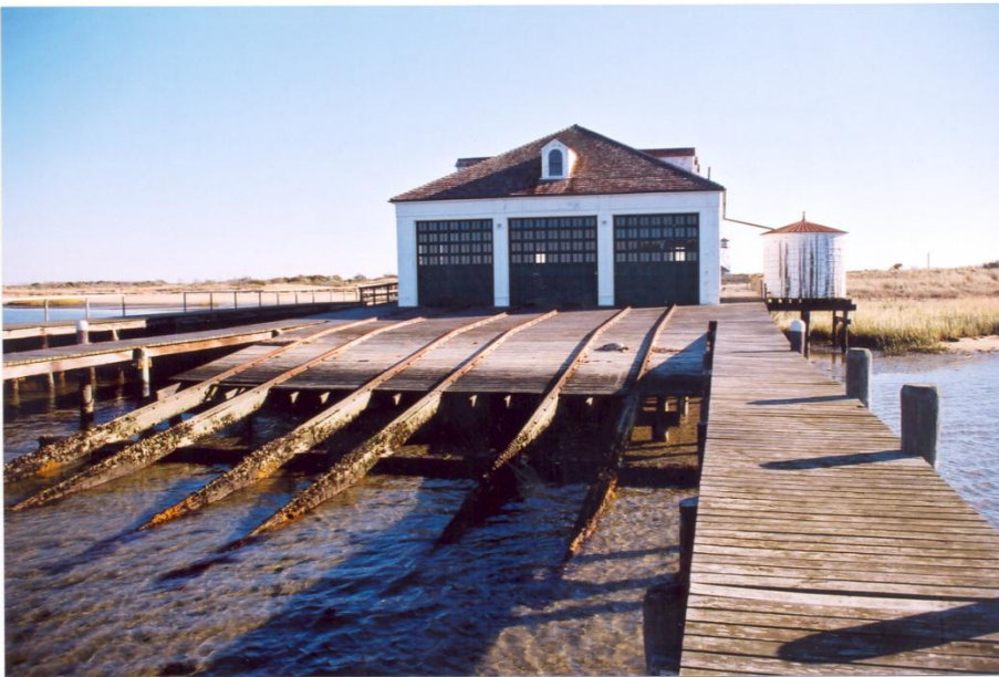
Figure 8. The boathouse and dock of the historic Assateague Coast Guard Station on Toms Cove Spit, Virginia. Image from Phillips (2007).
