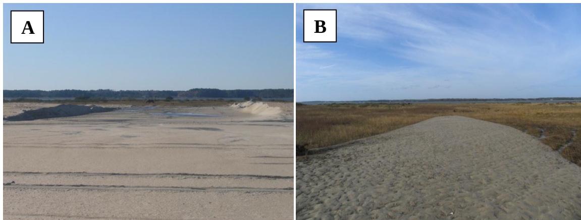
Figure 12. The constructed foredune was modified to restore overwash processes. A) Notches were dug in 2008 and 2009. B) As of 2011, the notches continued to allow overwash during storm events. Images from Assateague Island National Seashore.
