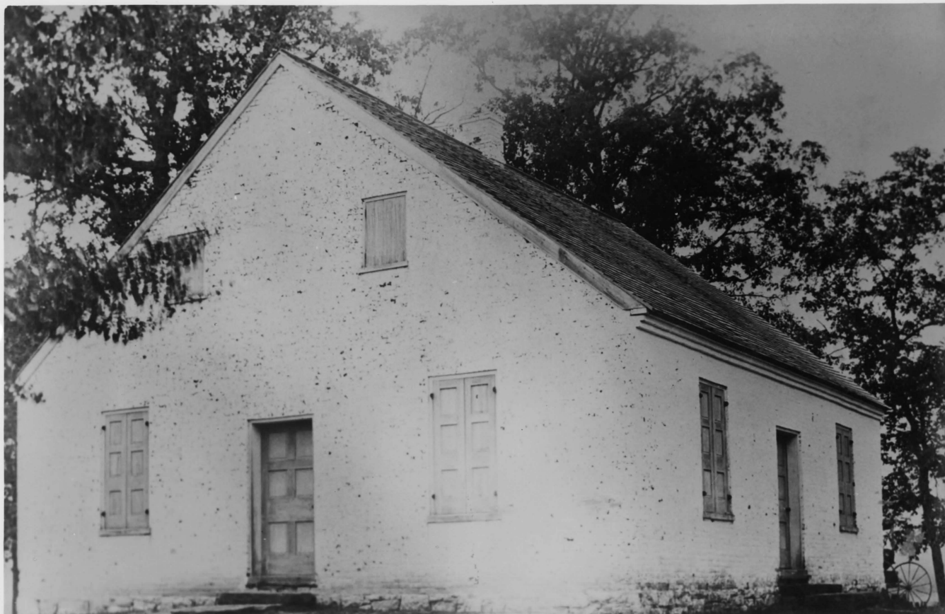
Photograph No. 7. The Dunkard Church, after the battle damage had been repaired. Exact date unknown; between 1864 and 1885. South and east walls are shown.
