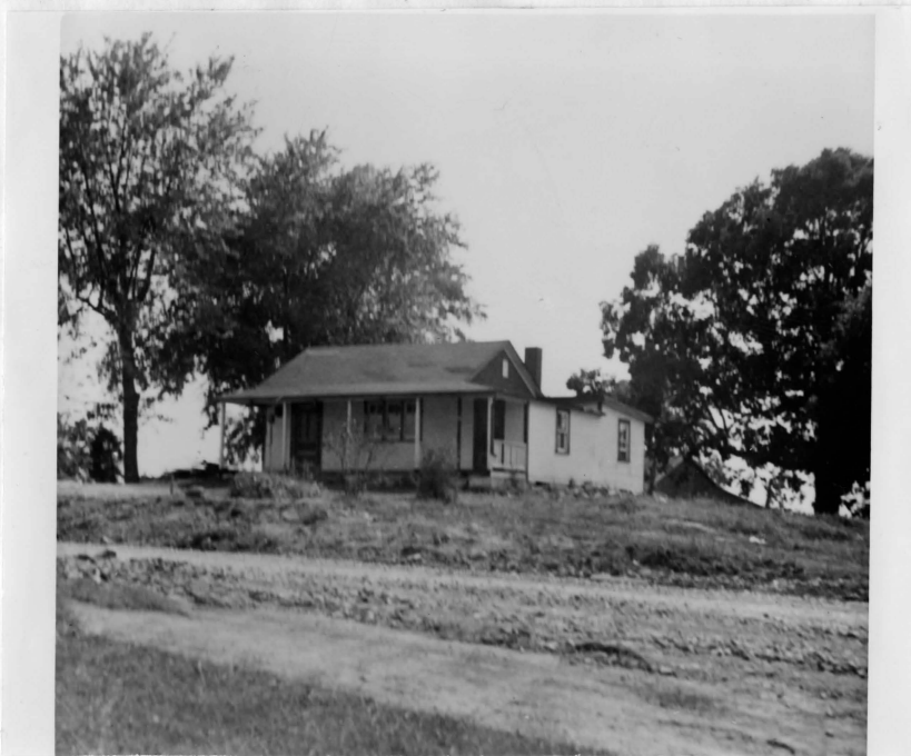
Photograph No.10. The frame dwelling erected on the Dunkard Church foundation in 1928, and occupied until 1951.
