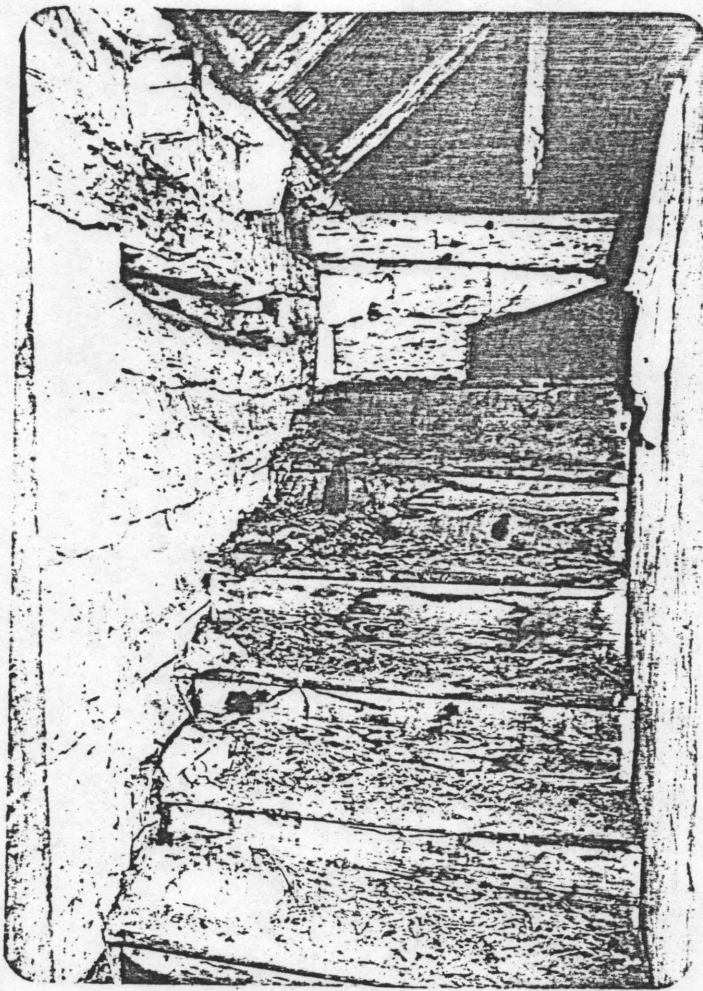
Photograph 9 Stairs to attic
