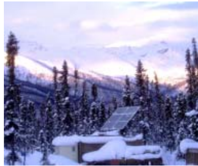
The new solar array sits atop the generator shed, providing power to the residences and ranger station throughout the summer months.
