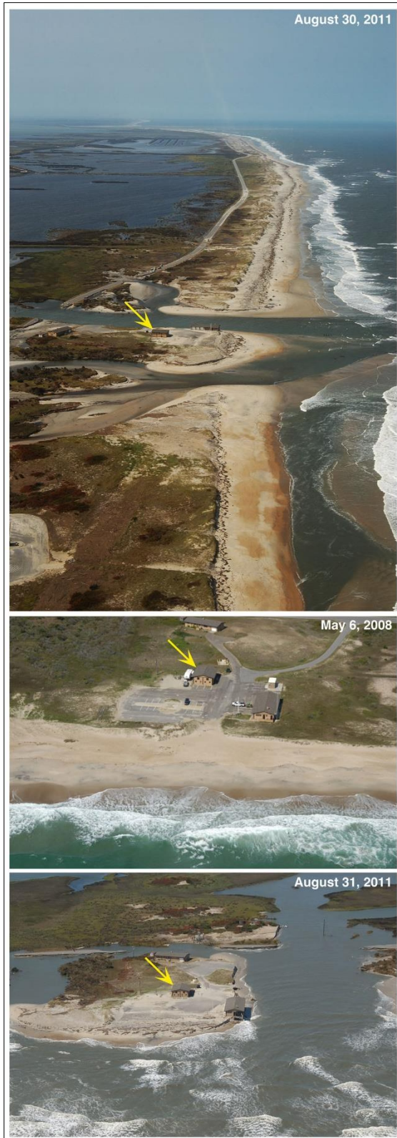
Figure 9. Pictures from pre- and post-Hurricane Irene on coastal North Carolina showing the breaching and land loss that occurred (USGS 2014).
