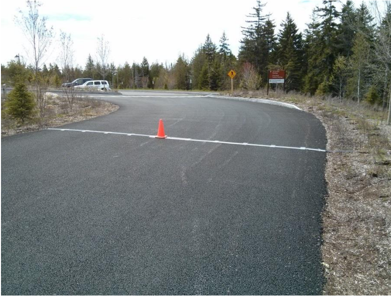
Day Use Parking Area: Traffic Counter secured to tree on right side of road.
