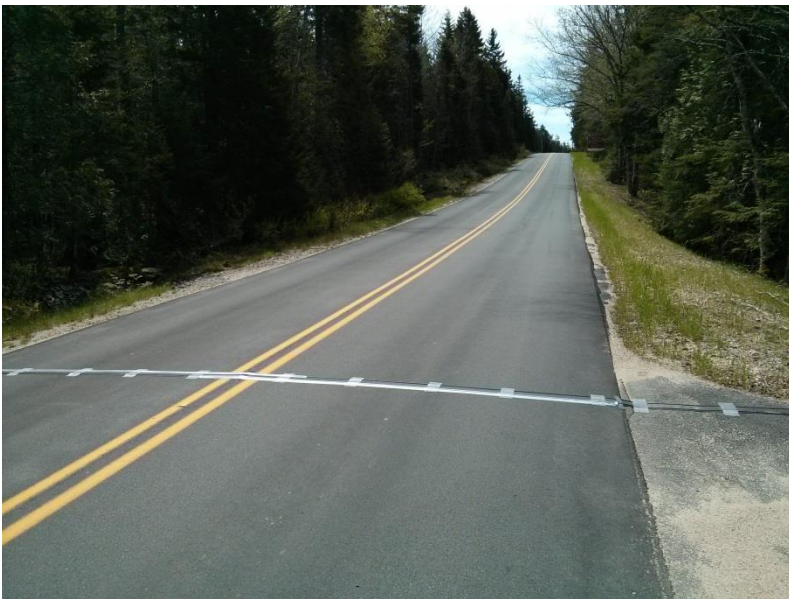
Schoodic Loop Road: Looking south. Traffic counter secured to tree on right side. Location is a utility vault pulloff.
