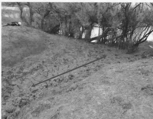
PHOTO NUMBER: 3 PHOTO DIRECTION: NE DESCRIPTION: Inlet/outlet to stockpond.
