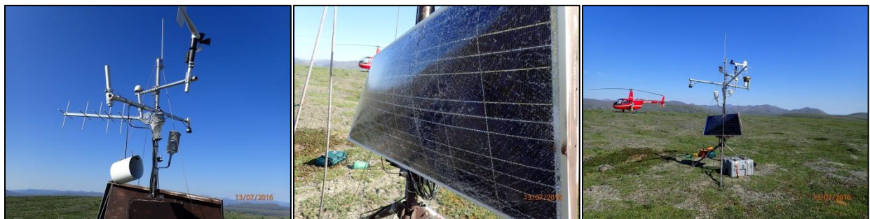
Figure 9. Sisiak climate station, July 12, 2016. Upon arrival at the site the crossarms were out of level, the tipping bucket was dangling, and the solar panel was damaged (left, middle). Site after maintenance (right). Note that the solar panel pictured was replaced on July 14, 2016.
