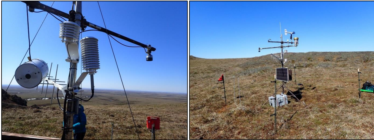
Figure 2. Devil Mountain climate station, June 1, 2016 before (left) and after (right) maintenance and repairs.
