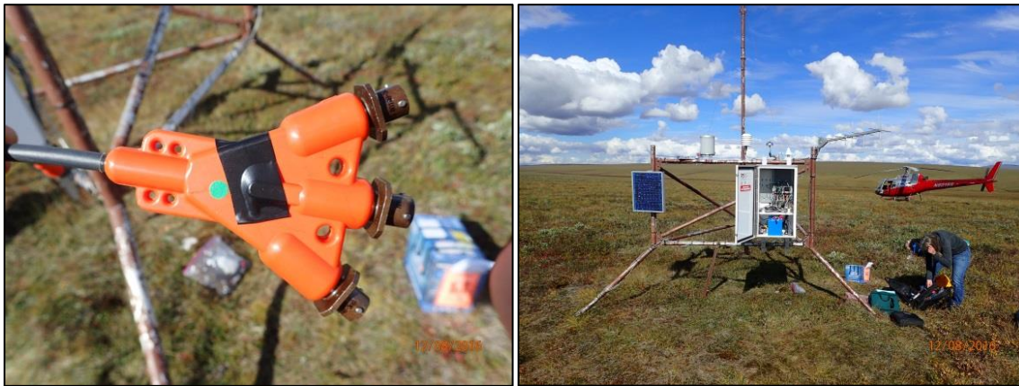
Figure 24. Noatak fire RAWS station, August 12, 2016 showing the damaged SDI expansion port that needs to be replaced at the next site visit (left) and the station after maintenance and repairs (right).
