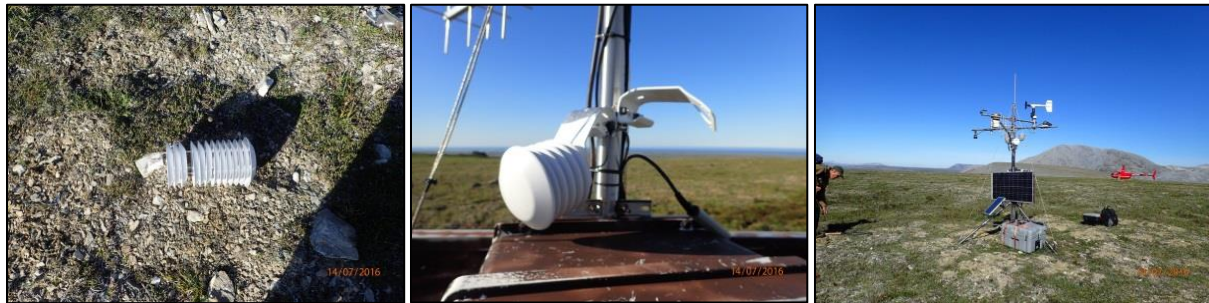
Figure 13. Mt. Noak climate station, July 14, 2016. The AT-RH sensor and shield were damaged and on the ground upon arrival (left). The radiation shield for the ThermX sensor (middle) was bent horizontally and not replaced in 2016. Photo after maintenance (right).
