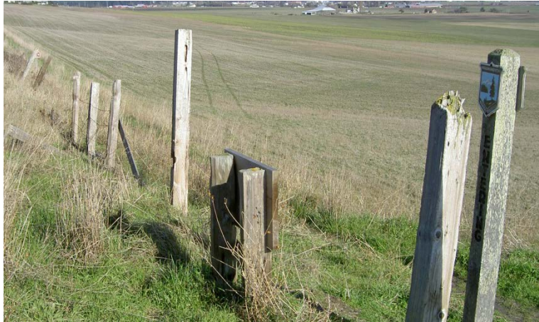
Figure 2. Leaning and Rotted Fence Posts
