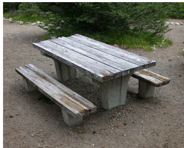
Figure 7. Picnic Table with Deteriorated Wood Surface
