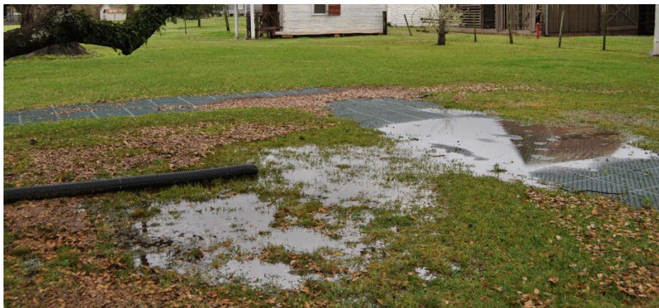
Figure 20. Ponding/Poor Drainage
