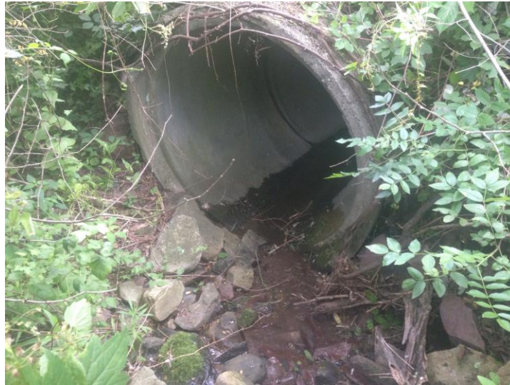
Photograph 4 – Unnamed tributary to the Upper Delaware River (R3UB1) view is northwest looking downstream at the section of the waterway as it passes through an RCP underneath Old Mine Road. June 2017 – P. Sharpe. (Photo Location Map – Appendix A)
