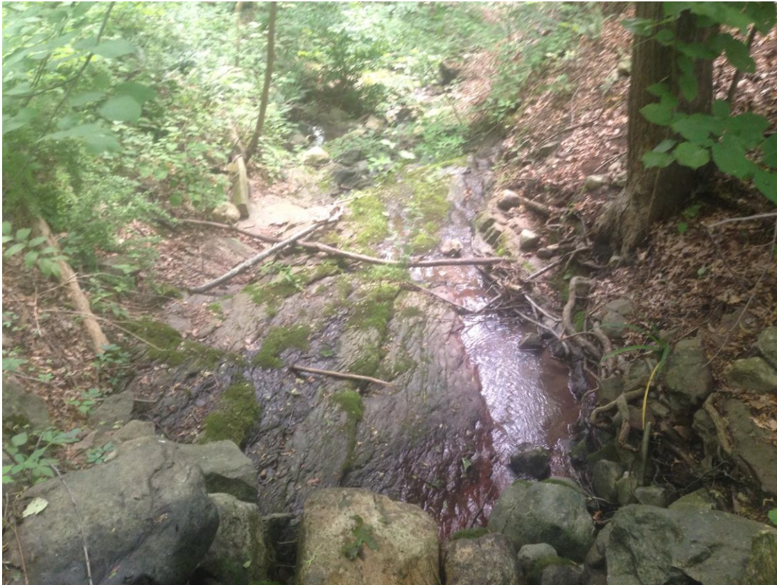
Photograph 5 – Unnamed tributary to the Upper Delaware River (R3UB1) view is northwest looking out of the RCP (downstream end) on Old Mine Road. Note the drop-off from the rock in the foreground to the waterway below. Photo taken June 2017 – P. Sharpe. (Photo Location Map – Appendix A)
