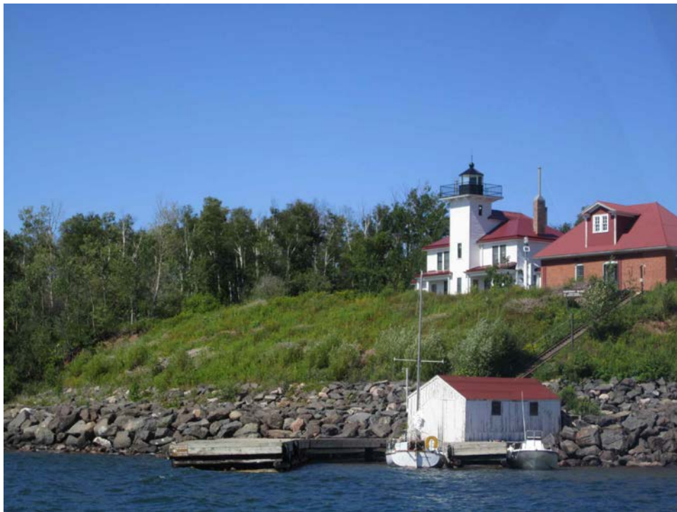
Figure 3. Shoreline stabilization at the lighthouse on Raspberry Island. View is to the north. Photograph is by Trista L. Thornberry-Ehrlich (Colorado State University).
