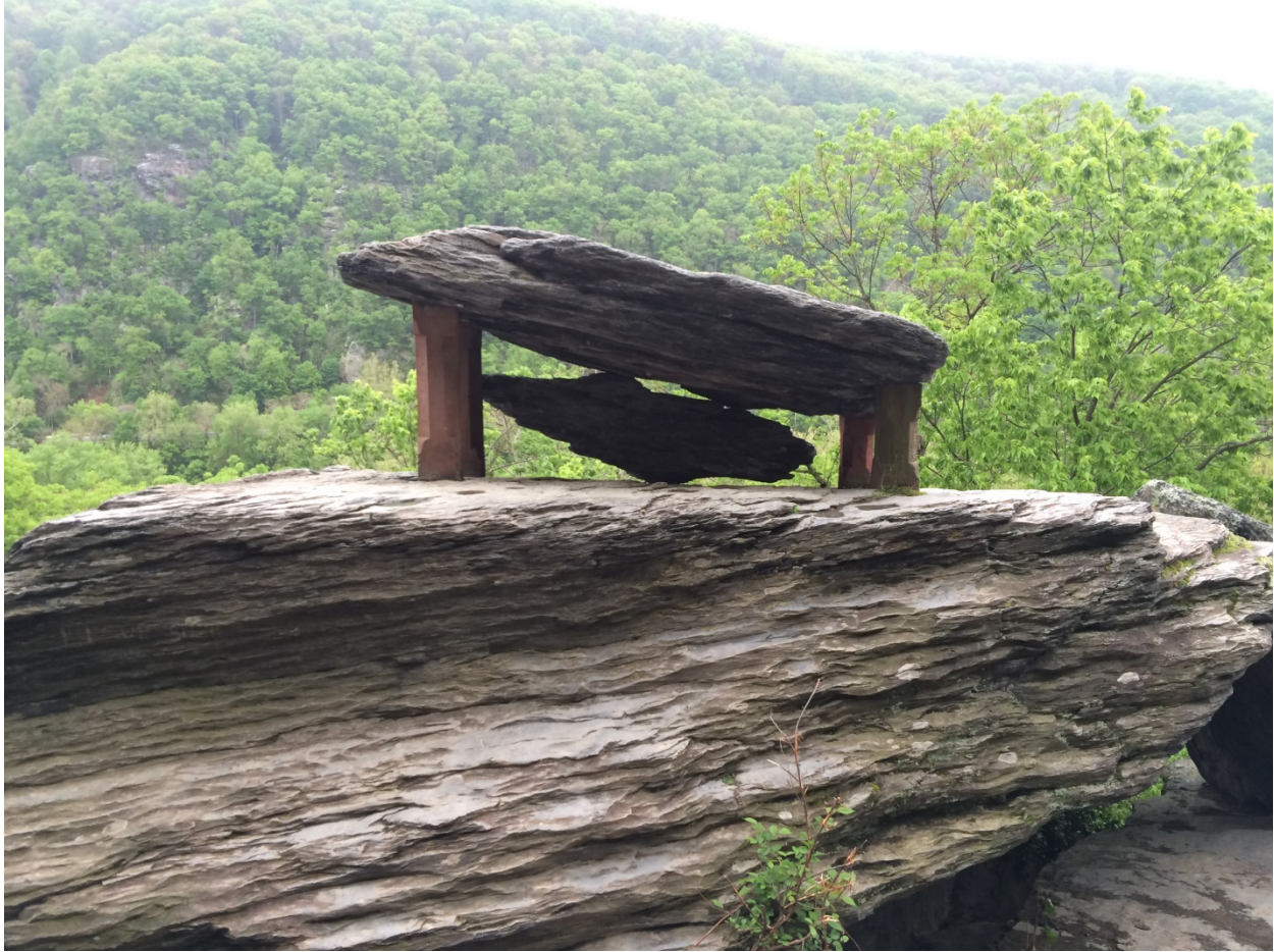
Figure 3. Photograph of Jefferson's Rock. Thomas Jefferson described the view of the Shenandoah and Potomac Rivers from this location in 1783. The supports were placed around the rock in 1860 to prevent it from falling. NPS photograph by Rebecca Port.
