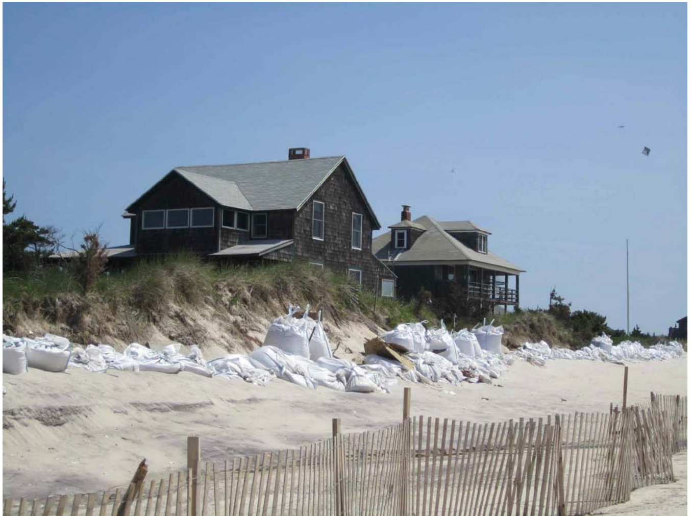
Figure 5. Houses at Point O'Woods with sandbags on the beach in an attempt to harden the seaward face of the foredune and reduce further erosion. Impact is associated with the March 2010 storm. View is to the northeast. Photograph is by Trista L. Thornberry-Ehrlich (Colorado State University).
