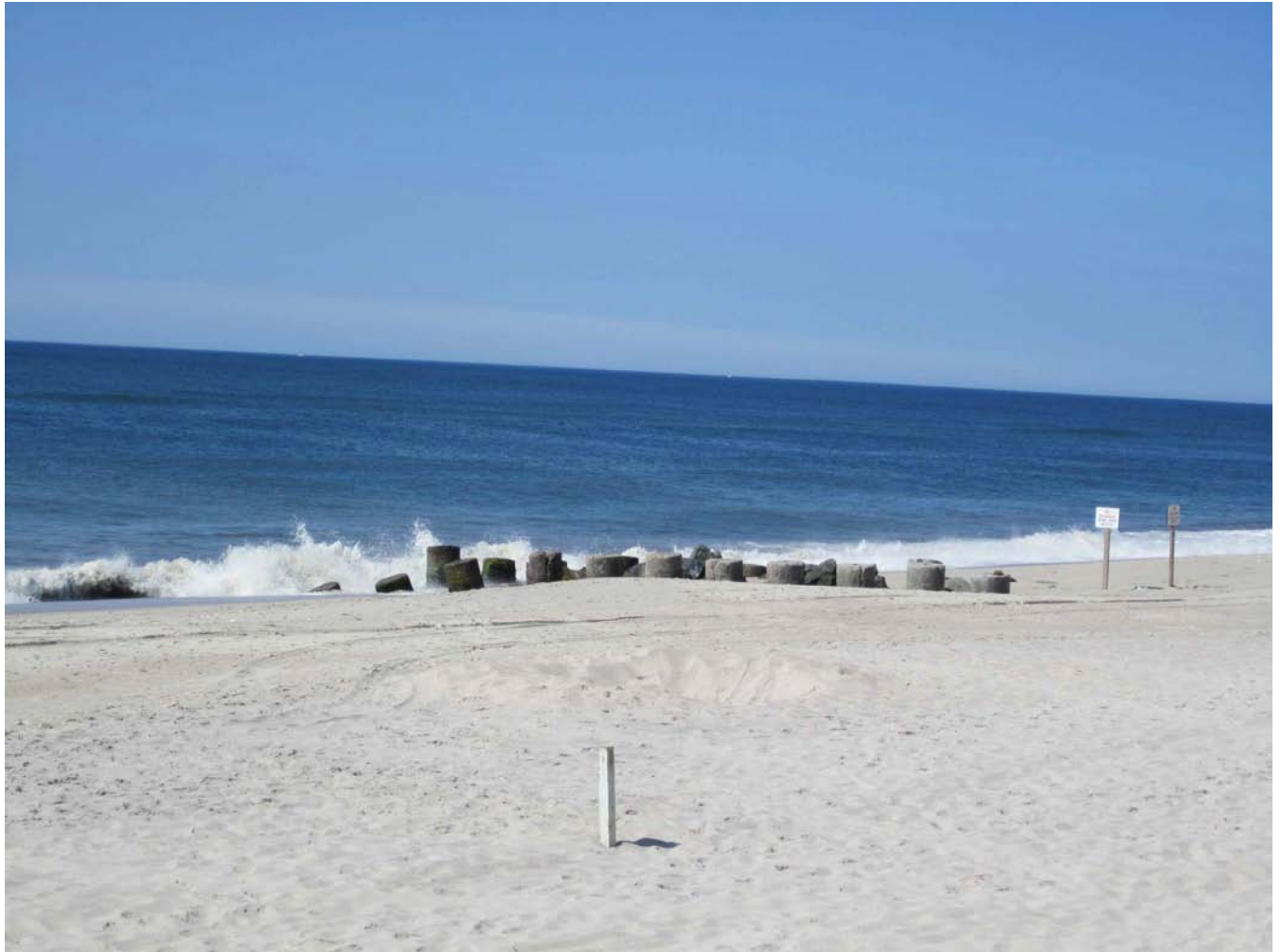
Figure 2. Groins at Ocean Beach. These tetrapods were originally put in place to protect a water tower from inundation and/or coastal erosion. The tower has since been moved inland. View is to the west. Photograph is by Trista L. Thornberry-Ehrlich (Colorado State University).
