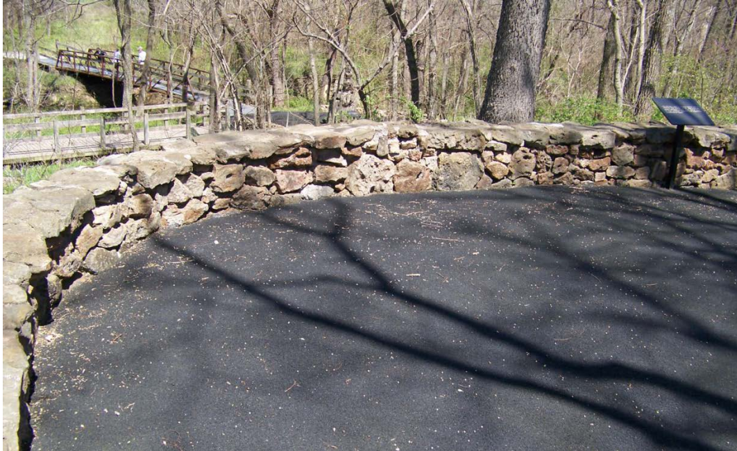
Figure 7. Rock walls, such as this one at Field Trip Stop 1, were constructed using local rock probably from either the Warsaw Formation or the Burlington-Keokuk Limestone. Photograph by John Graham (Colorado State University).
