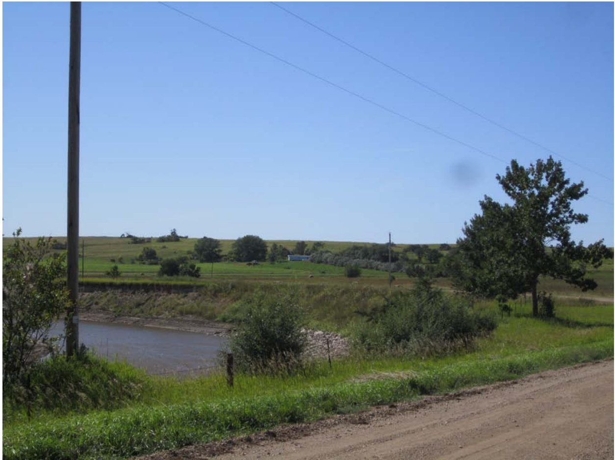
Figure 3. Steep cutbank along Knife River adjacent to a county road that traverses the park. Photograph by Trista L. Thornberry-Ehrlich (Colorado State University) August 16, 2011.
