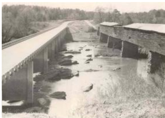
Figure 2. New bridge and old bridge. Alabama 49 runs through the northwestern part of Horseshoe Bend National Military Park. The Alabama-49 bridge crosses over the Tallapoosa River. Miller covered bridge once provided access over the river. Construction of the present-day bridge was completed in 1956. The covered bridge collapsed in 1963, a year after this photograph was taken. Base support structures of the covered bridge remain. Photograph (right) by Katie KellerLynn (Colorado State University). National Park Service photograph (left, ca. 1962) available at http://www.nps.gov/hobe/photosmultimedia/Miller-Covered-Bridge.htm (accessed November 2, 2012).
