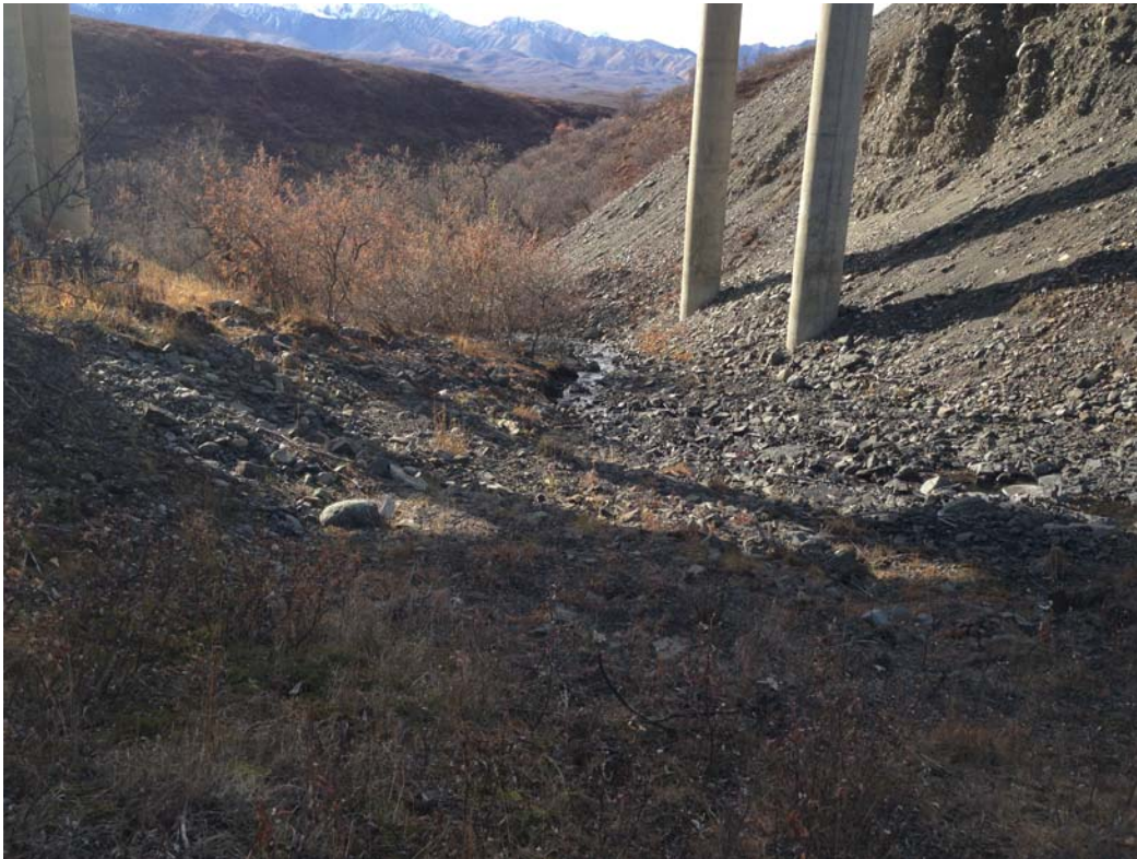
Photograph 1. Photo looking south at the mapped riverine wetland feature and a pair of the existing bridge supports of the Ghiglione Bridge at DENA. September 2017
