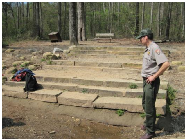
Figure 7. Steps near Devils Race Course Shoals. The steps, which provide river access, are losing support as a result of fluvial erosion exacerbated by sudden water release from Burford Dam. Photograph by Katie KellerLynn (Colorado State University).
