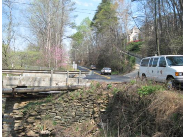
Figure 5. Sloped driveway at Sope Creek. During storms, this driveway near Sope Creek becomes a spillway for storm-water runoff. Photograph by Katie KellerLynn (Colorado State University).
