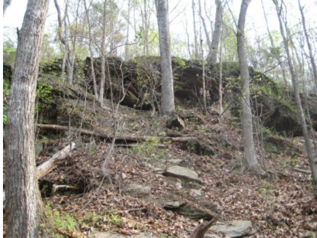
Figure 17. Rock shelter. The rock shelter shown in the photograph occurs near the Chattahoochee River at Island Ford Shoals. It is the result of weathering of crystalline bedrock. Photograph by Georgia Hybels (NPS Geologic Resources Division).
