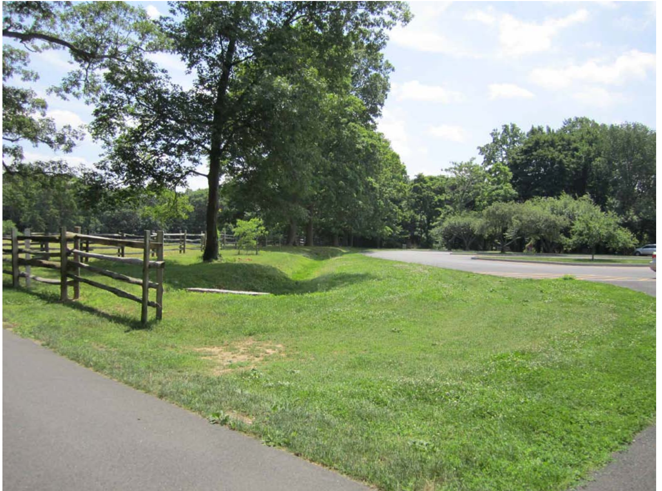
Figure 9. Drainage ditch channeling runoff from park's main parking area to the perennial kettle. View is to the south, the kettle sits north of the view point. Photograph is by Trista L. Thornberry-Ehrlich (Colorado State University).
