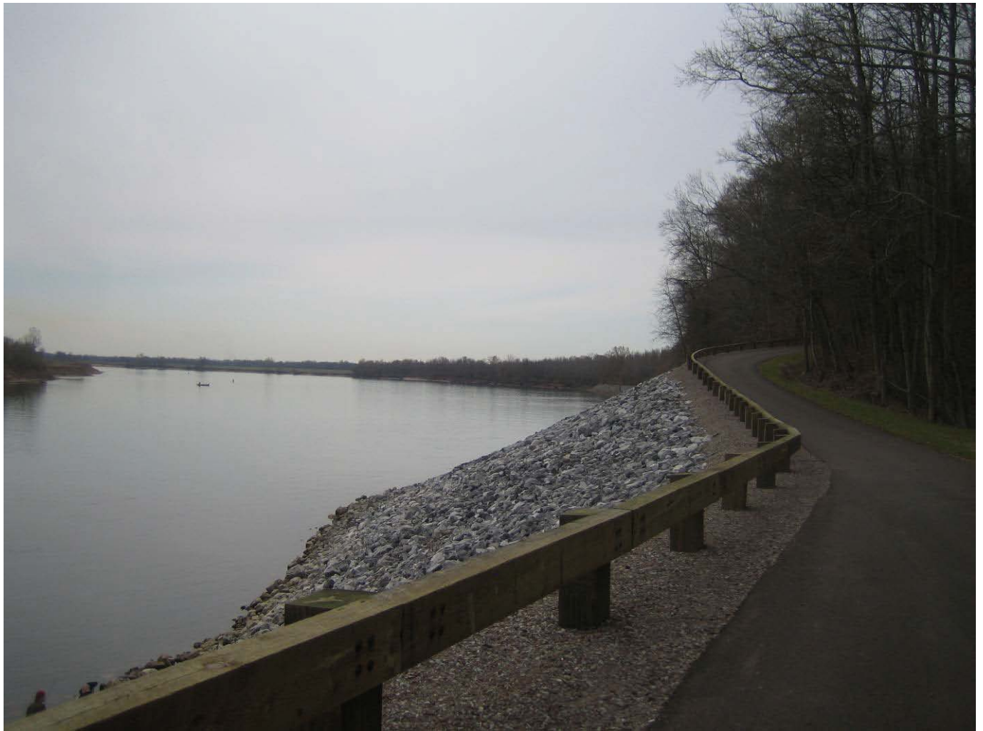
Figure 2. Limestone armoring the Tennessee River shoreline at Shiloh National Military Park along Riverside Road. Photograph is by Trista L. Thornberry-Ehrlich (Colorado State University).
