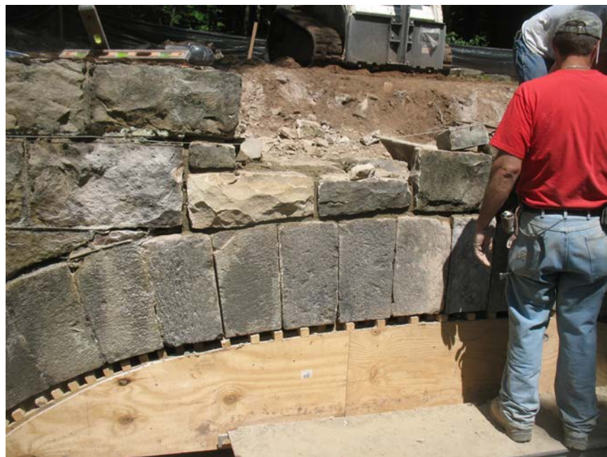
Fig. 4 Wall being rebuilt
