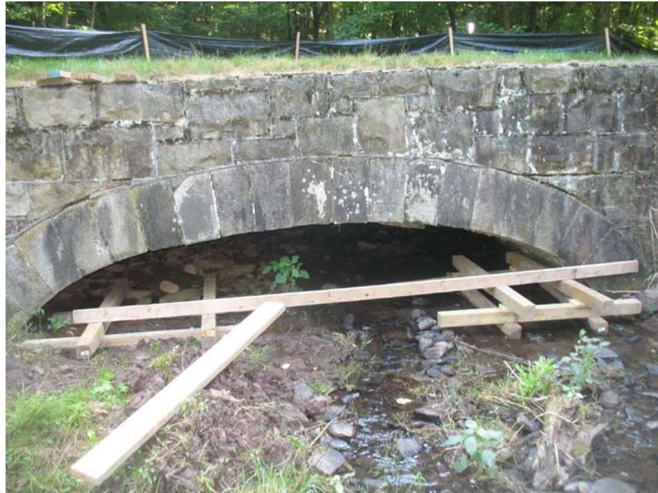
Fig. 1 Cribbing for centering being levelled
