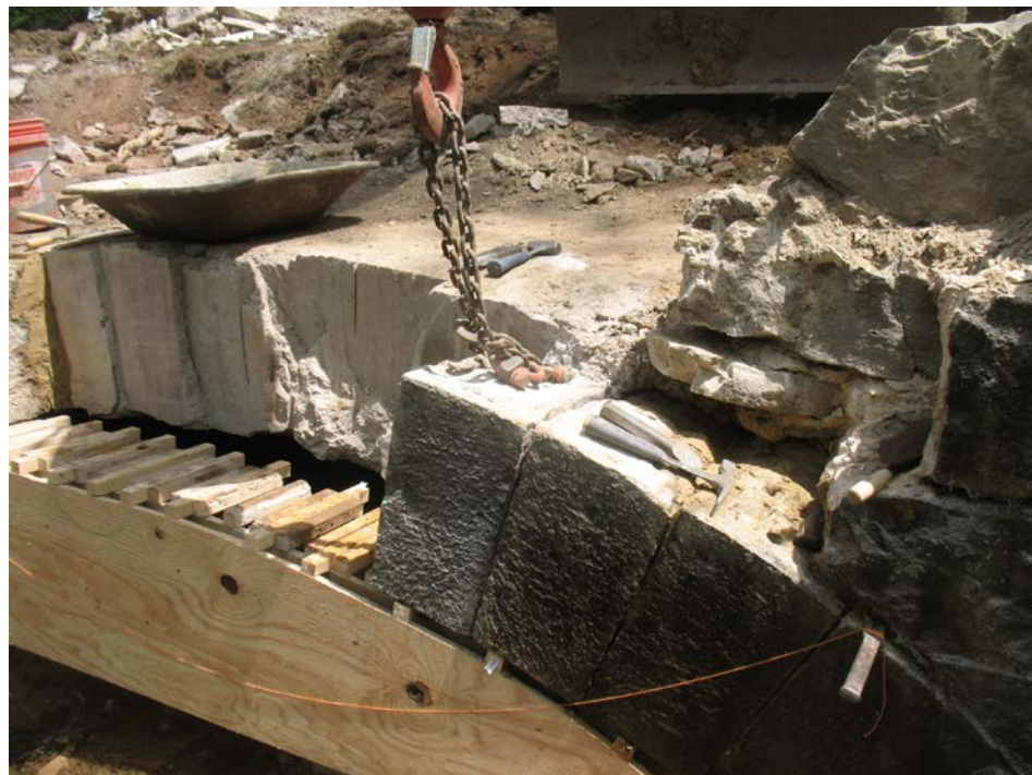
Fig.2 Resetting ring stones
