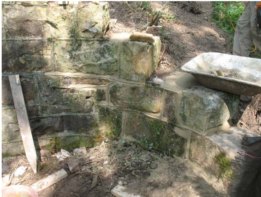
Fig.5 Rebuilt wing wall section
