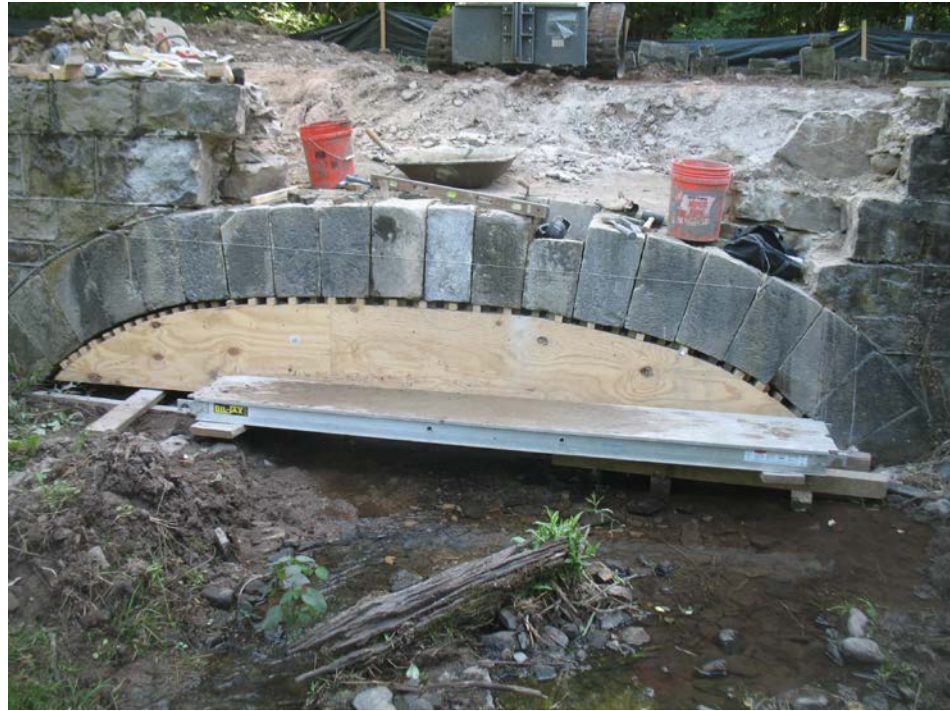
Fig.3 Ring stones reset
