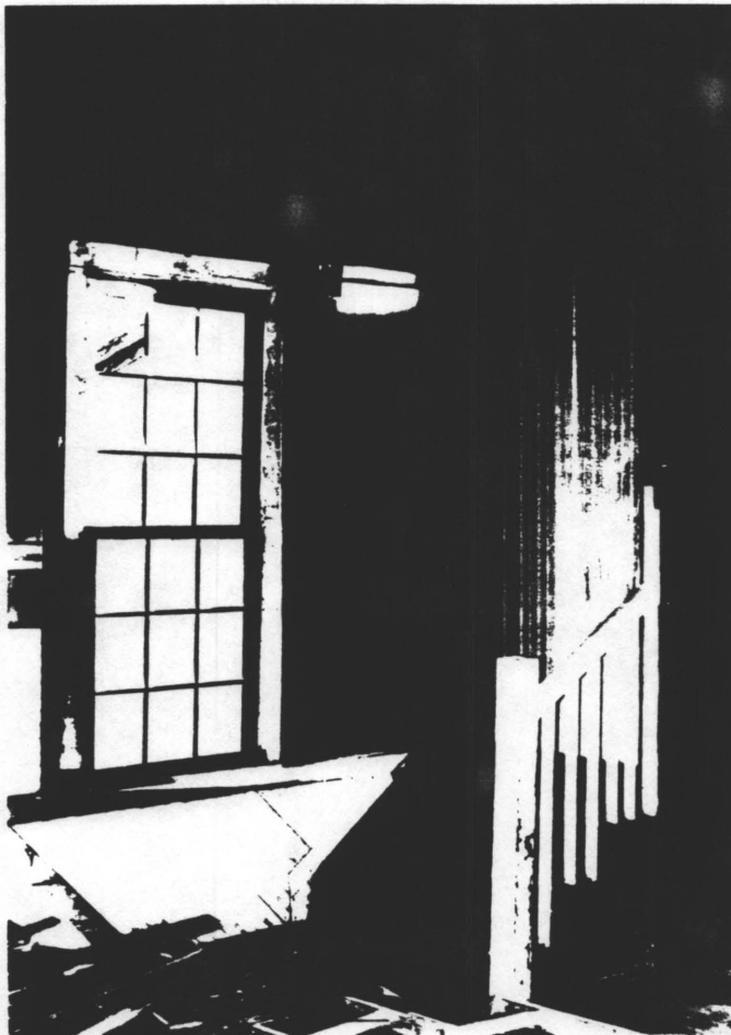
PHOTOGRAPH 24 ORIGINAL CABIN, EXISTING STAIRCASE IN NORTHEAST CORNER.
