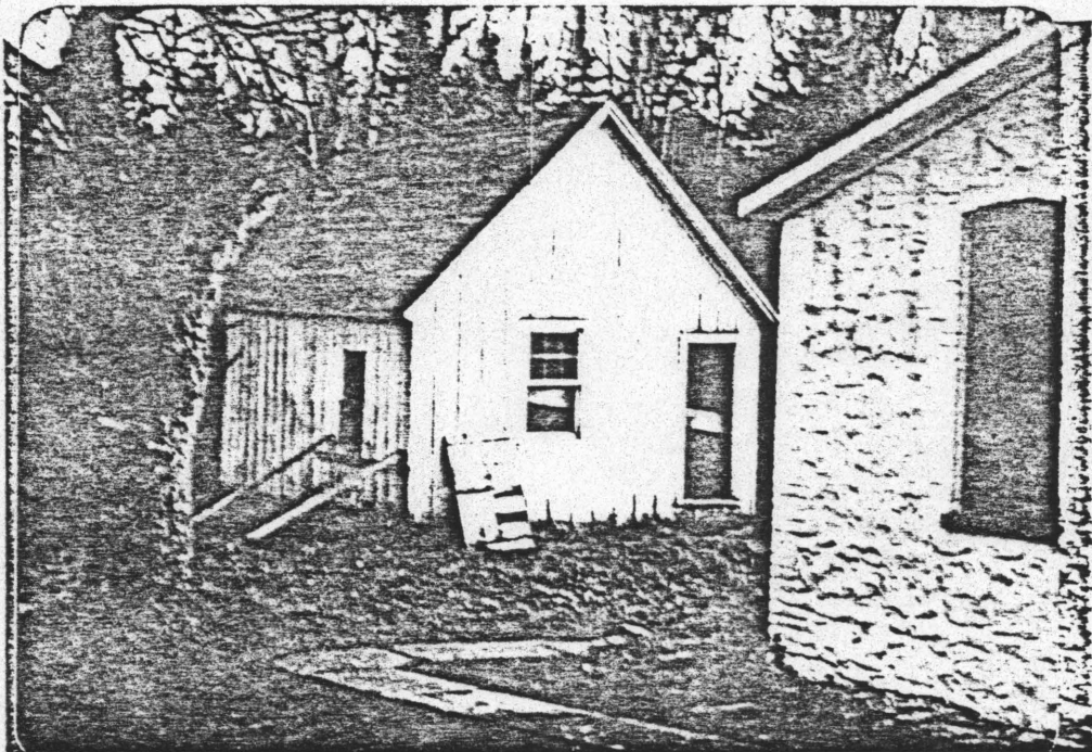
Photo showing storage shed HS-23-103B. Structure had been raised to prevent further deterioration to siding and frame work. Interior and exterior had been temporarily braced.
