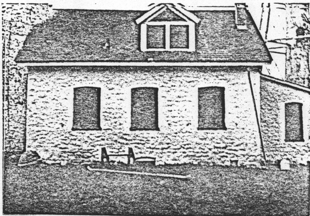
Photo shows east side of Lighthouse after whitewash was applied. Temporary shutters were constructed for all windows and door openings.
