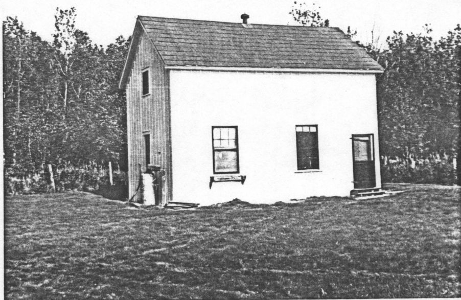
20), Photo shows work on the first quarter resident completed.
