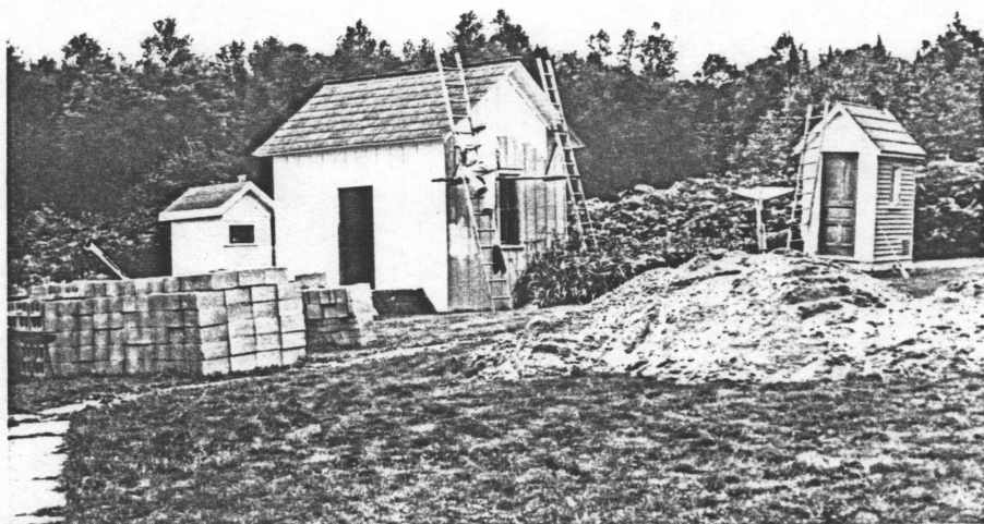
16) Photo showing primer being applied to the shed HS-08-102F. The building to the left is Privy HS-08-102E and to the right the small privy HS-08-102D.
