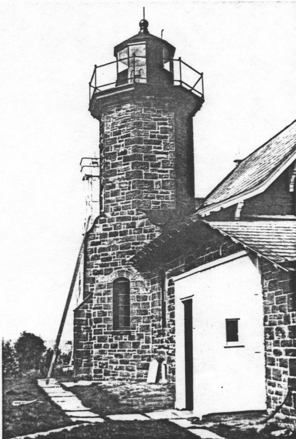
10) Southwest view showing lighthouse stabilization work near completion.
