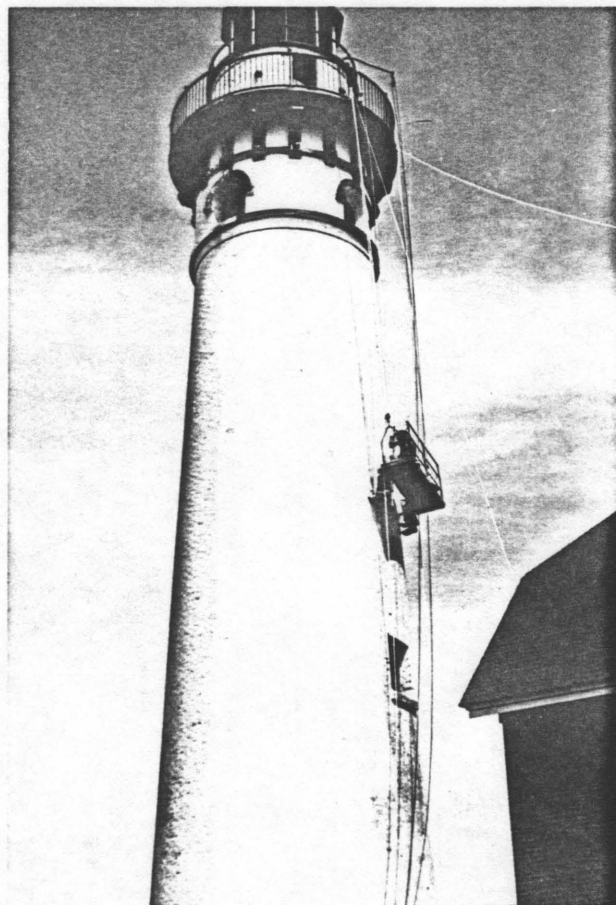
Decorative trim has been painted and workmen proceeding in the white-washing of the tower.
