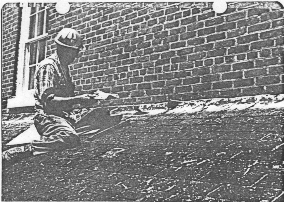
New flashing being installed along lean-to section over kitchen wing (south side).
