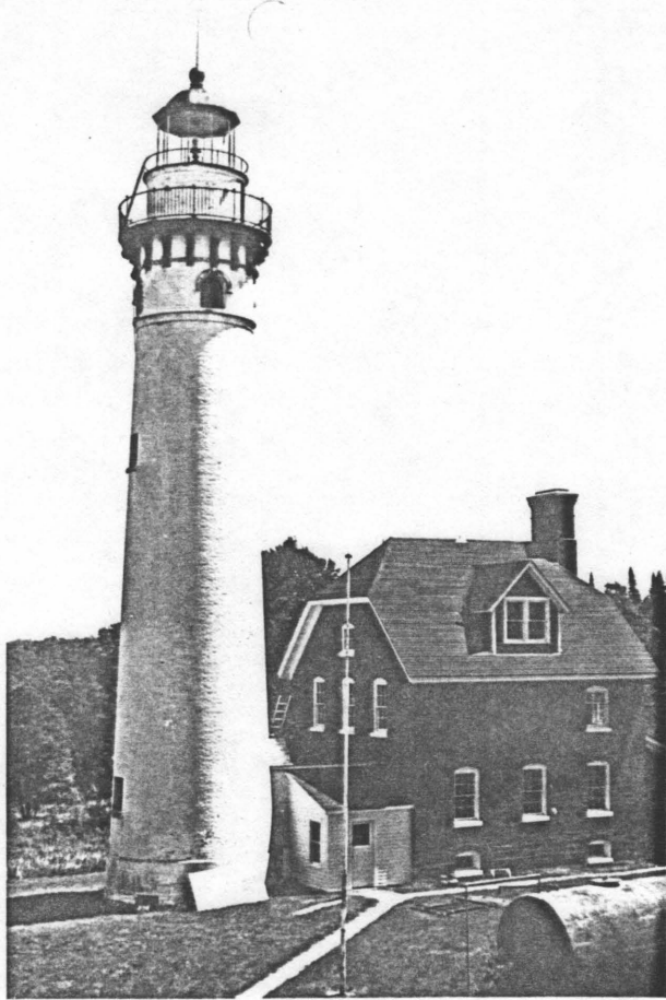
Northwest view of the lighthouse during one of the construction stages. Majority of the work had been completed on the house.
