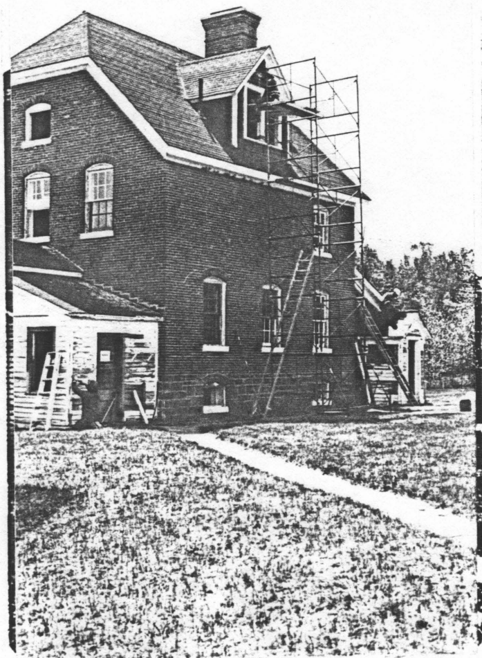
Workman preparing the lighthouse for painting, HS-22-105A.
