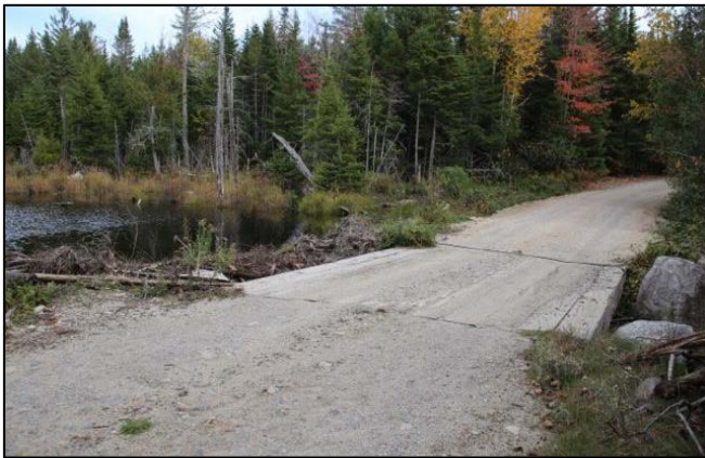
Photo 2: Entrance to Loop Road Bridge and Beaver Dam
