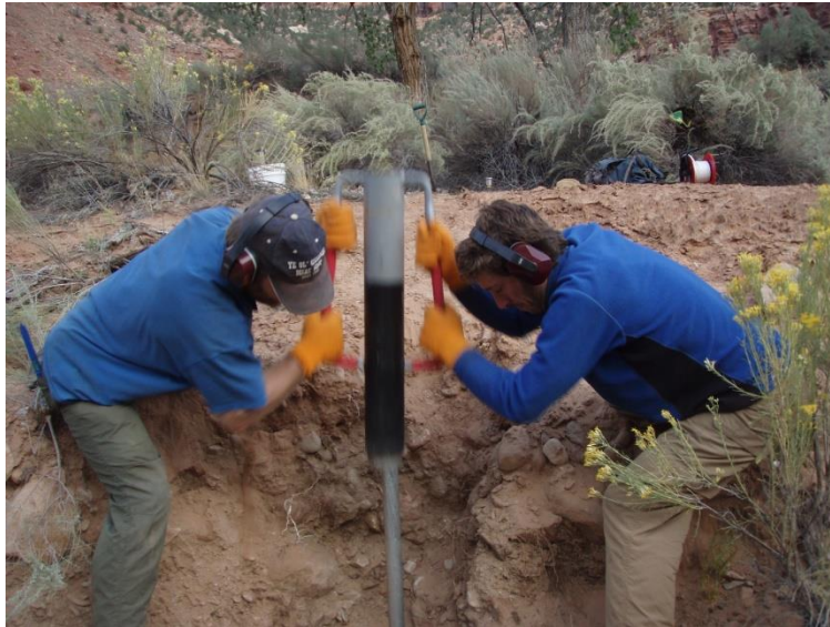
Figure 4. Installing a riparian well at the East Fork of the Virgin River, Zion National Park.
