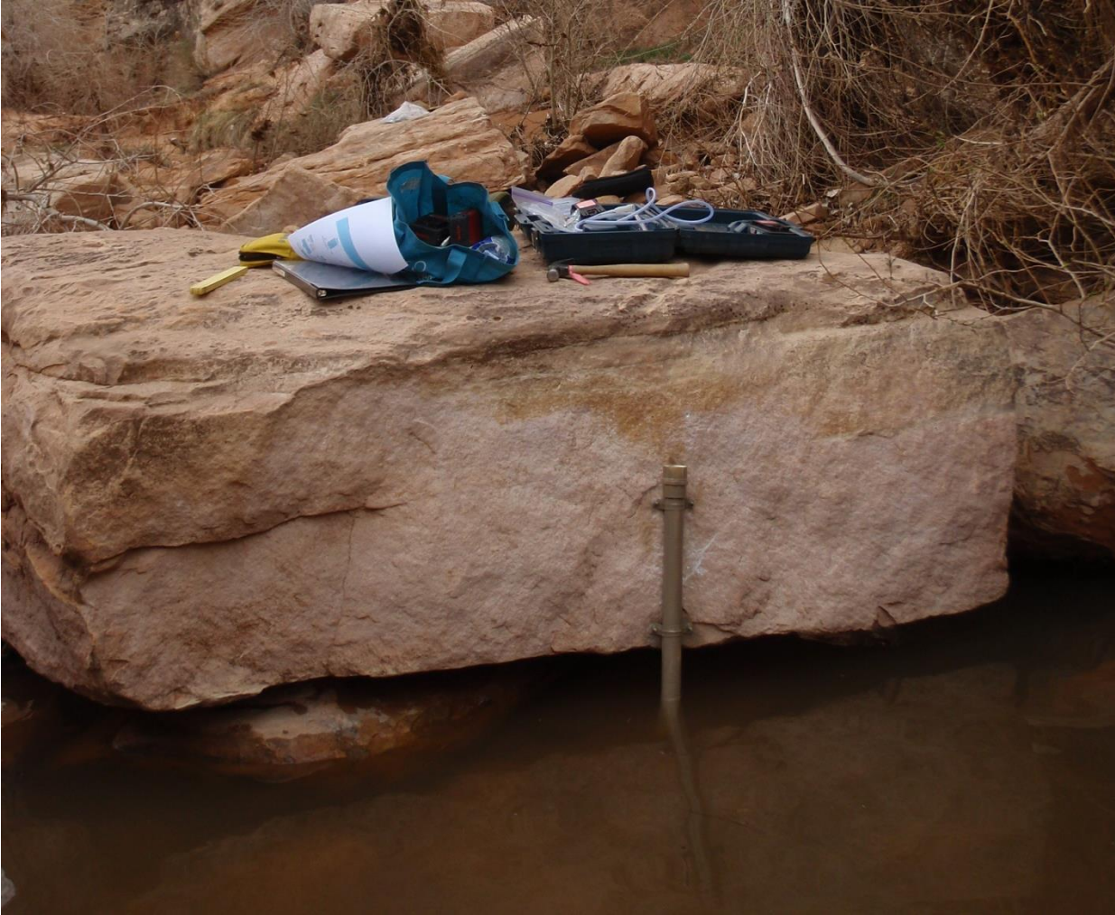
Figure 9. PVC casing instream installation at Natural Bridges National Monument.
