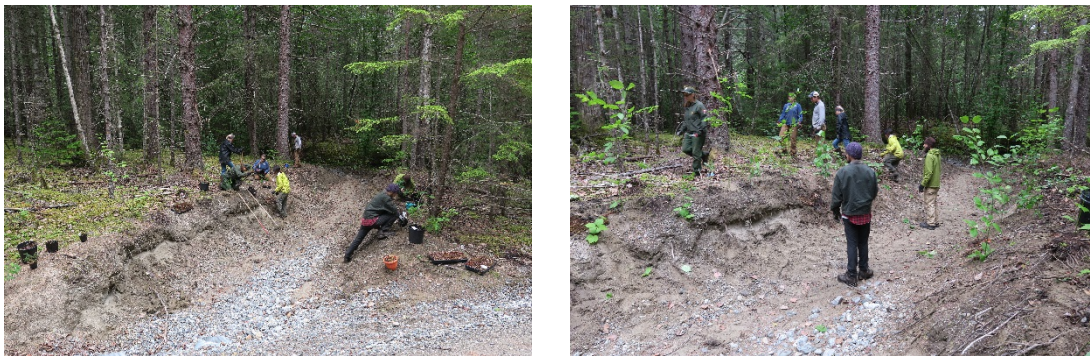
Figure 22. The culvert site before (left) and after (right) restoration
