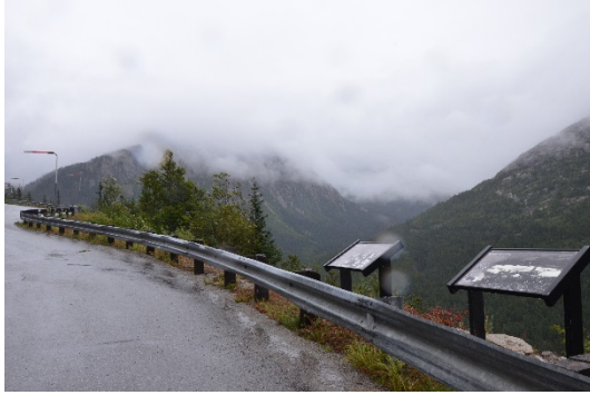
Figure 30. The ground past the Dead Horse Gulch overlook's guardrails is infested with many invasive plant species.
