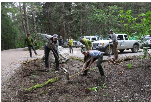
Restoration work at Slide Cemetery
