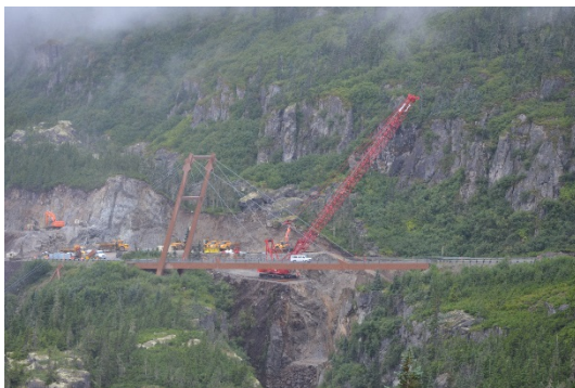
Figure 31. Construction of a new bridge to replace the Captain William Moore Bridge will pose a large disturbed area when finished.
