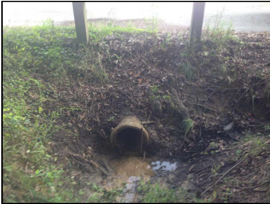
Photograph 4 (P4) – 12 inch RCP which serves as the only visible outlet for the 85.52 acre watershed system draining to this point. View is northwest August 2017 – P. Sharpe.
