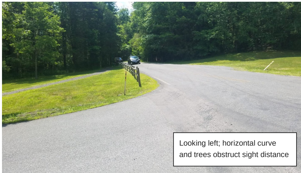
FIGURE 3-6: INSUFFICIENT INTERSECTION SIGHT DISTANCE LOOKING FROM PARK HEADQUARTERS ONTO RIVER ROAD
