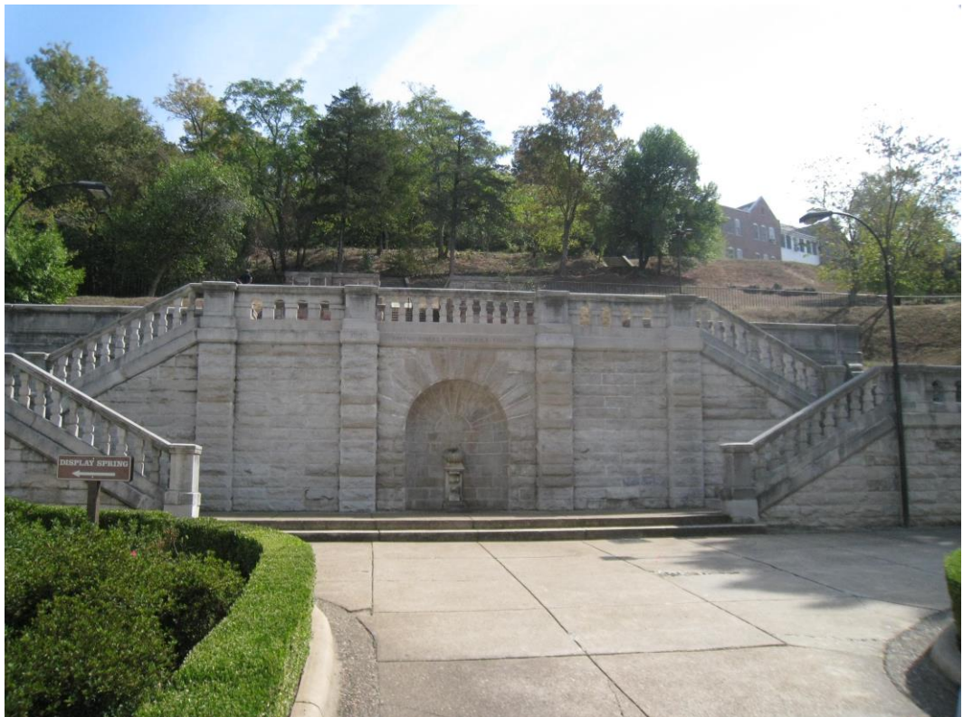
FIGURE 10: MAIN ENTRANCE TO THE GRAND PROMENADE
