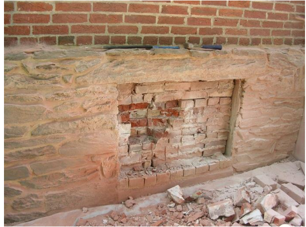
Figure 2 : Some of the window openings had been bricked over. Here, the HPTC wood crafting team begins to open up one of these window openings.
