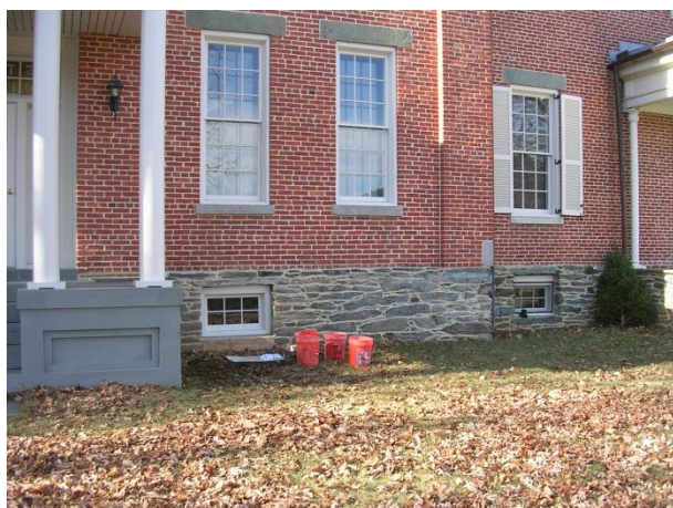
Figure 5 : A completed sash installation
