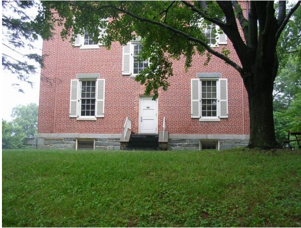
Figure 7 : The HPTC wood crafting team also worked on the doorways of the Wirth Hall. Pictured above is a doorway that has been wet scraped and sanded to remove any flaking or failing paint; primed with Benjamin Moore alkyd primer; wiped down with deglosser; and painted with Benjamin Moore semi-gloss latex paint to matching the existing paint.
