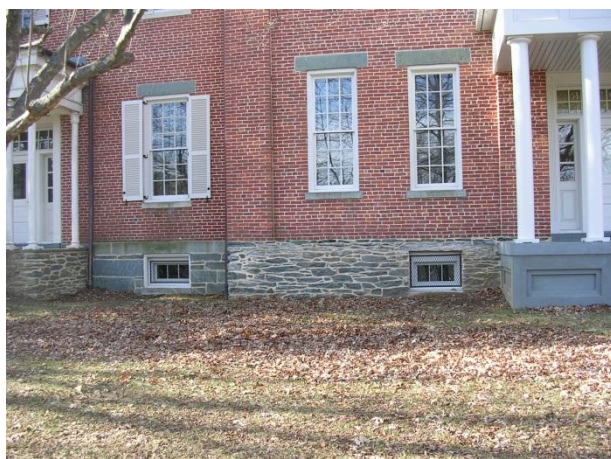
Figure 6 : Final window unit repairs. Once the window units were replaced, the stainless steel mesh panels were reinstalled.
