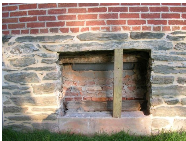
Figure 3 : When opened, four to five layers of brick courses were discovered. Whole bricks were saved and given to park maintenance; the remaining debris was disposed of.
