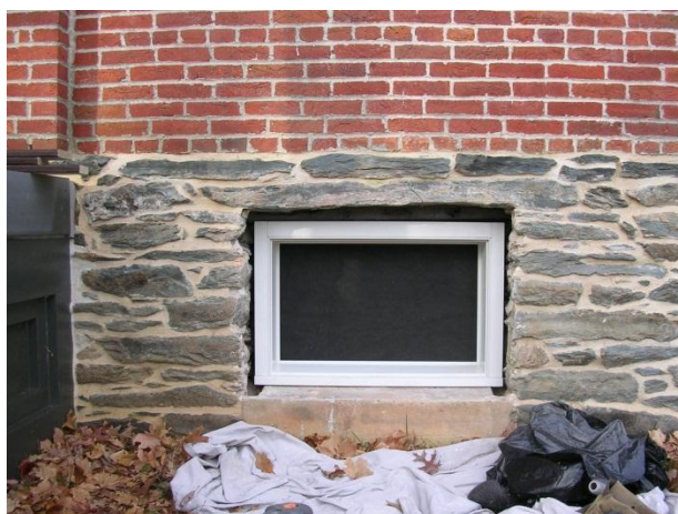
Figure 4 : The window sash were taken to HPTC's Jenkins shop facility for abatement and repairs before being reinstalled in their respective openings. Above, a repaired sash is reinstalled.
