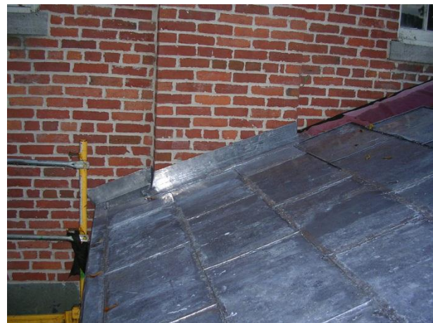
Figure 10 : The starter strip was attached to the eaves and rake edges with copper nails. The lead coated copper pans were fitted together and nailed with clips on the two edges that were not mechanically locked. The pans were then soldered together, with the ridge being folded over and soldered.
