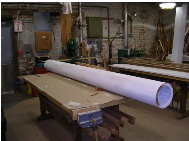
Figure 9 : After they were machined to a smooth round column, the columns were sanded, and primed with oil based primer on the inside and outside.
