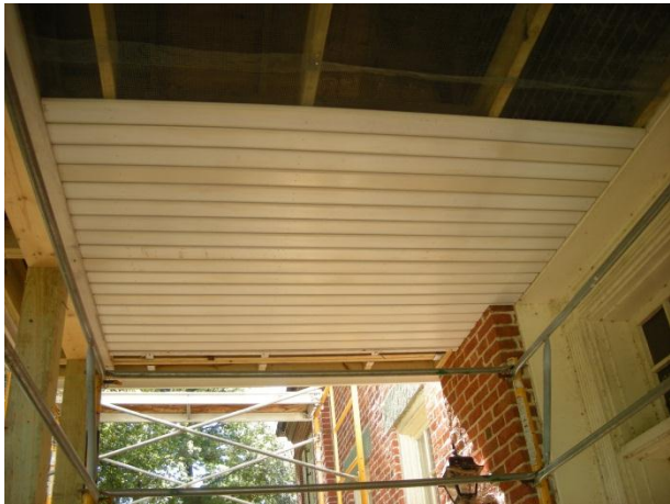
Figure 7 : The crew installed the double beaded ceiling boards with 1/4" spacing between the boards.
