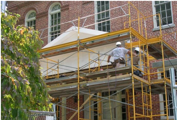
Figure 5 : The architrave was installed with the 3 mahogany wood panels being attached to the framing followed by the 8" wide frieze casing and the 6" wide vertical frieze trim. The installation of the frieze panel molding on the inside of the casing completed the fabrication of the architrave panels. The mahogany pediment panel was completed with the installation of flashing on the sill of the pediment and the installation of the frieze casing and panel trim inside the pediment.
