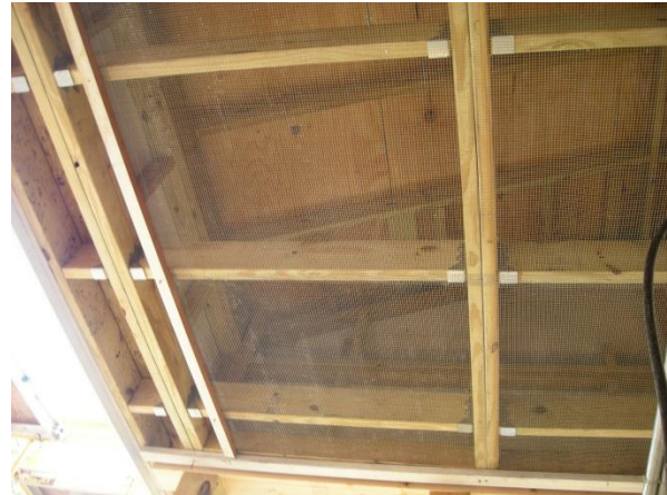
Figure 6 : Wire mesh was installed beneath the double beaded ceiling boards.
