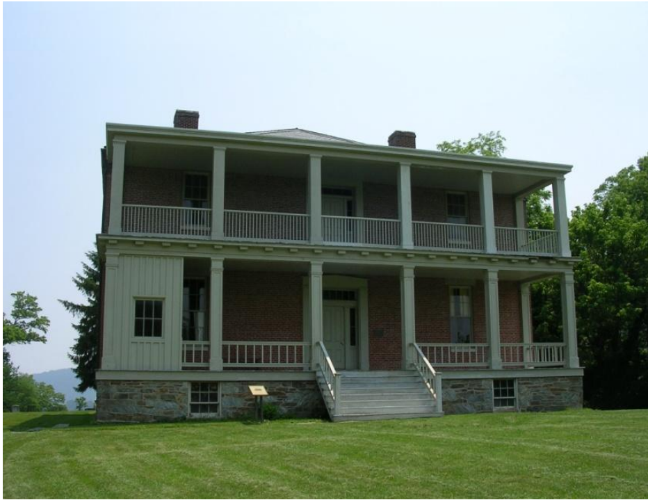
Photo #1- Lockwood House before preservation of the second story porch started in August.
