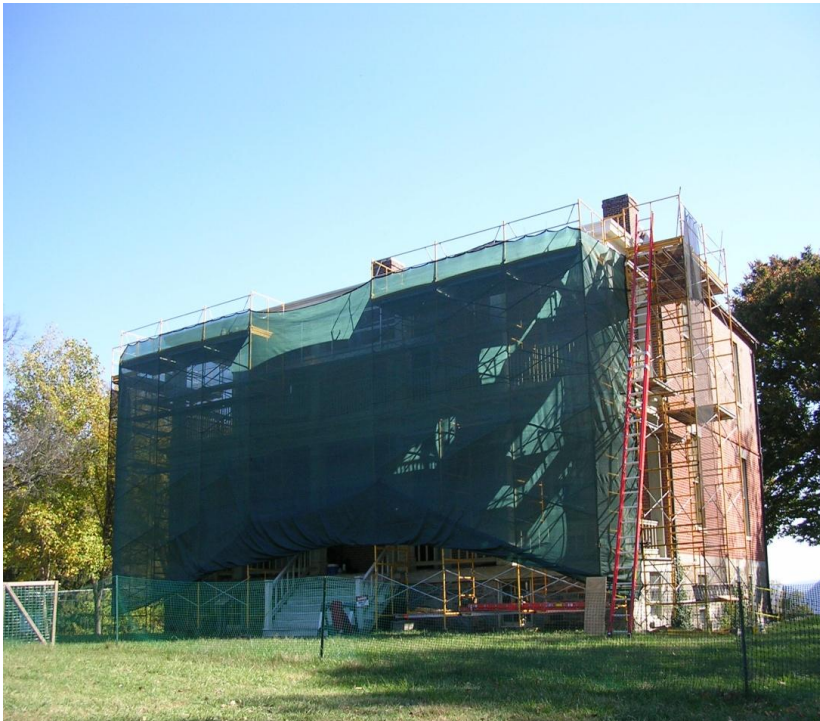
Photo 2: Scaffolding is erected around the perimeter of the west porch; shade cloth has been draped over the scaffolding.
