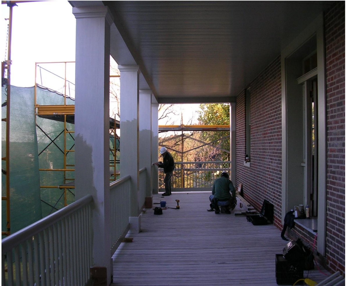
Photo 7: Porch flooring is being prepped for painting, columns are also being painted, and the base is being replaced with Spanish cedar material.
