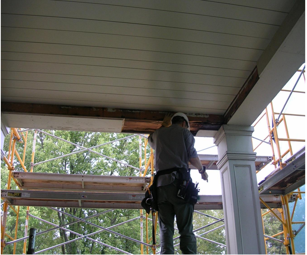
Photo #5- The breast beam trim is being replaced with new Spanish cedar trim and the ceiling boards have all been replaced with new Spanish cedar boards.
