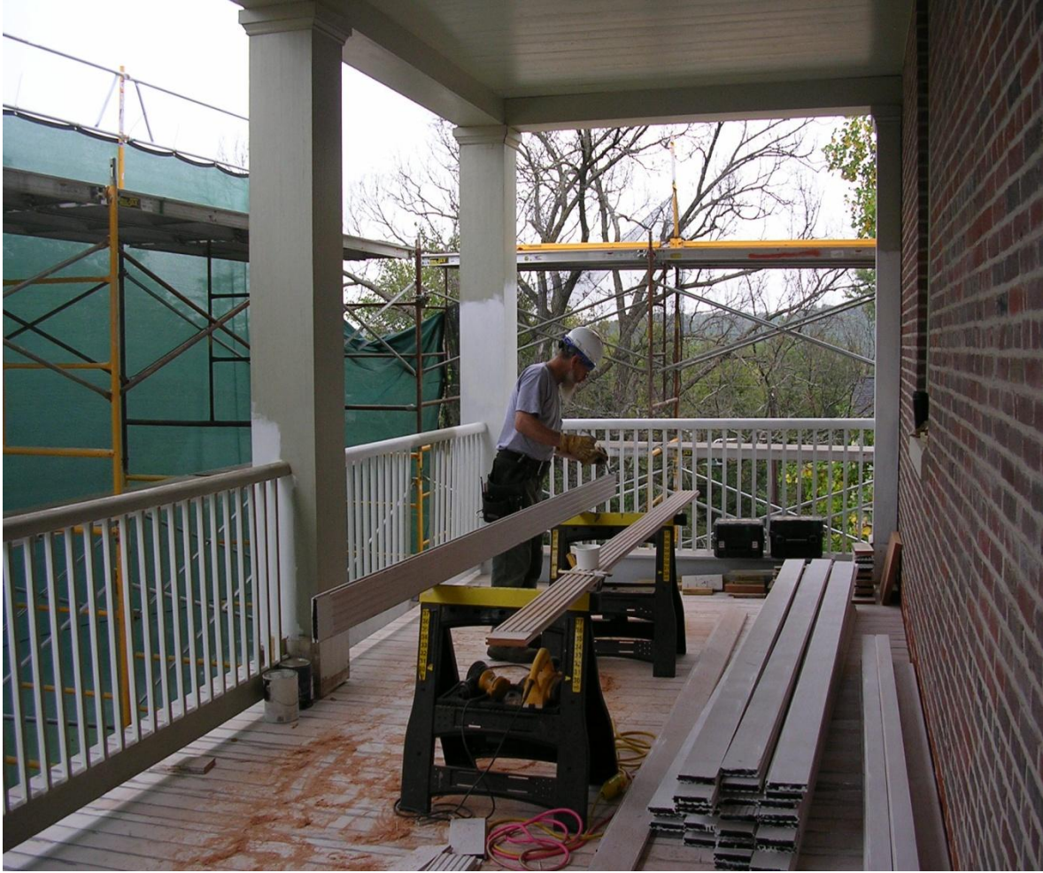
Photo 6: Photo shows the replacement flooring is being painted on the tongue and groove for maximum weather protection; it was then installed with historic cut nails.
