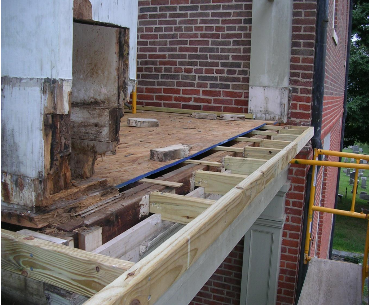
Photo #3- The framing for the architrave has been replaced with treated material; the picture also shows a deteriorated column, which was repaired.
