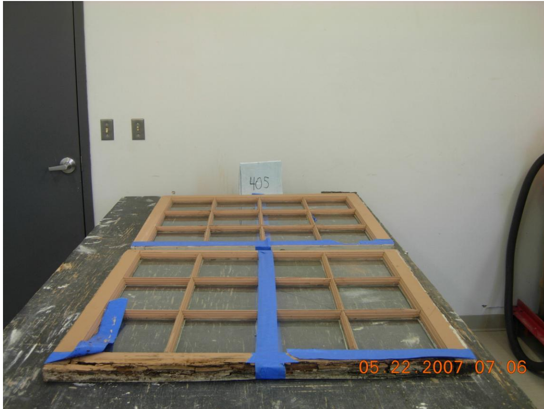
Photo 5: Deteriorated sash of building 35
