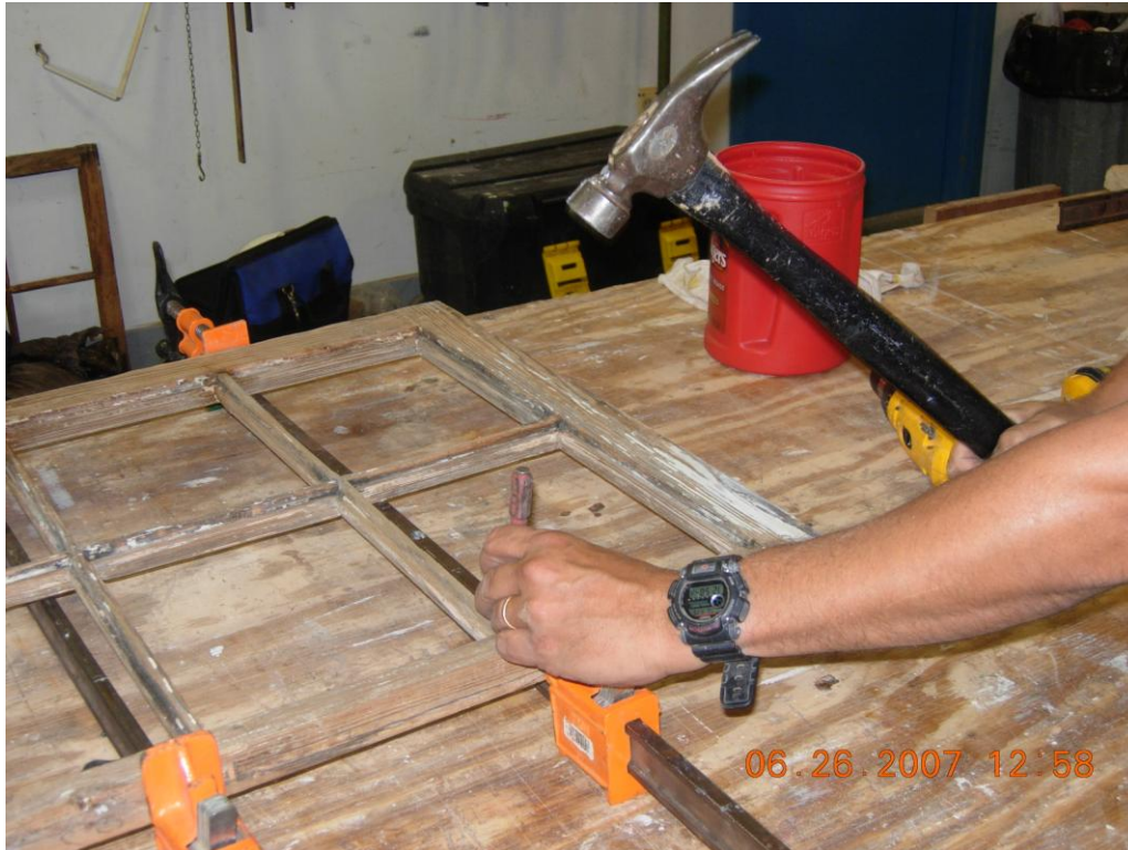
Photo 7: Sash repair in progress (setting new sash sprigs).
