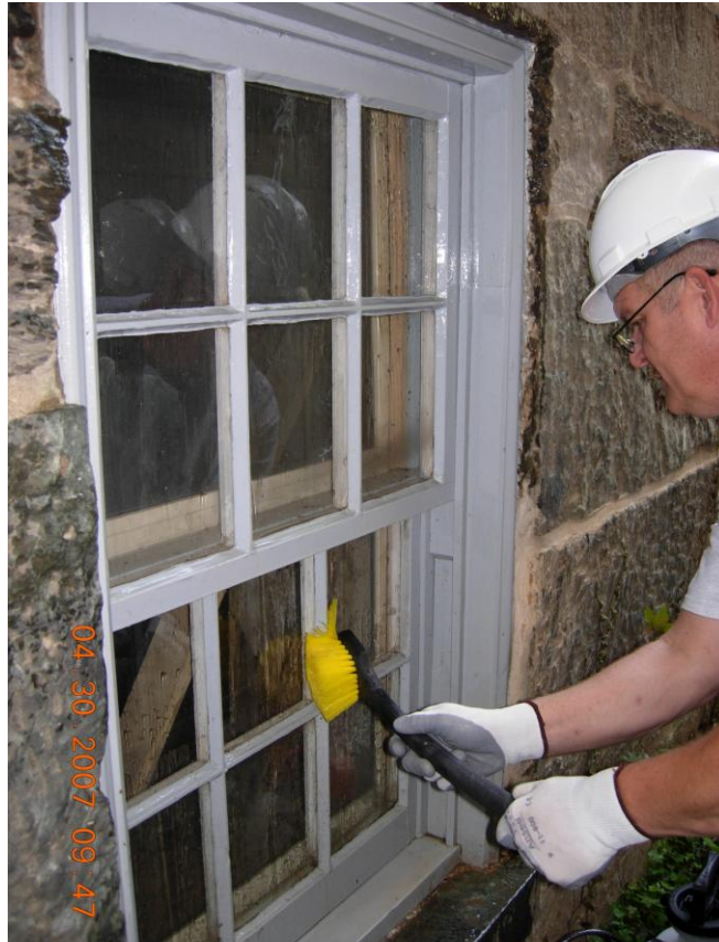
Photo 1: Cleaning procedures of basement level sash on Building 36
