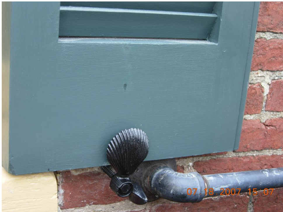
Photo 8: Preserved shutter hung with new clam shell shutter dog attached
