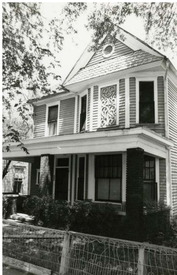
Figure 32. Undated (c. 1985) south facade of 526 Auburn Avenue prior to exterior improvements. Non-historic brick porch posts have not been removed in this photo. The photo also shows a fence on the southern property line.
