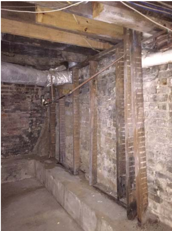
Figure 49. Southwest corner of basement.
