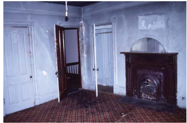
Figure 100. Office 202 oblique view toward north (MALU Archives, Slide 526_02, April 1985).
