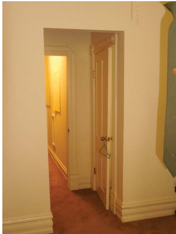
Figure 105. Office 204 view toward west.
