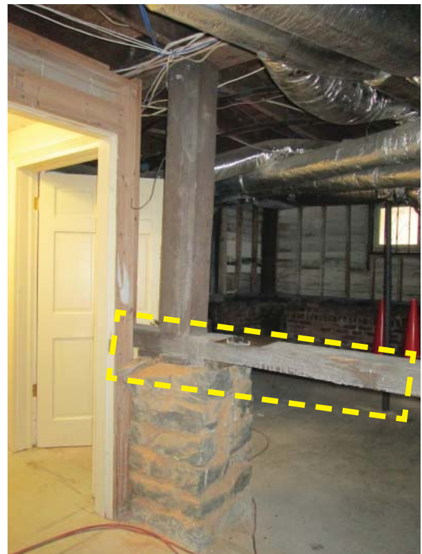
Figure 53. Wood support frame under bearing wall running North-South northern end. Low beam has been removed for door. Outline of area added for emphasis.
