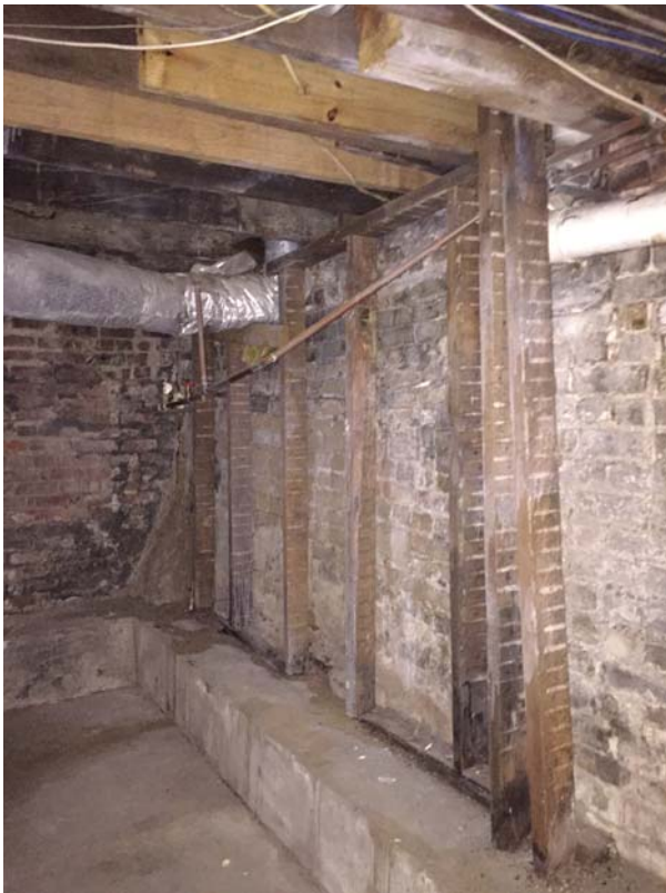
Figure 71. Unfinished Basement view toward southwest.
