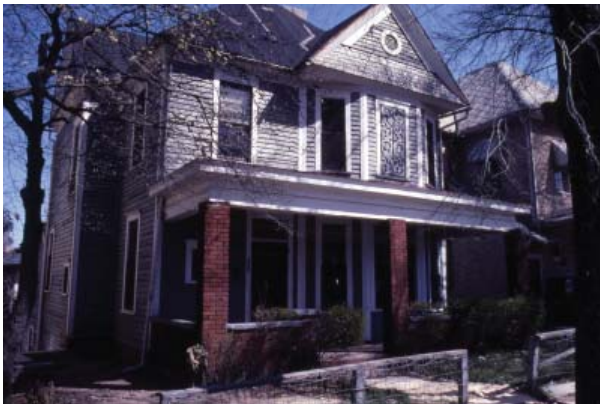
Figure 44. South elevation (MALU Archives, Slide 526879, March 1985)
