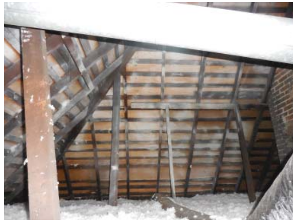
Figure 56. Roof framing in attic.
