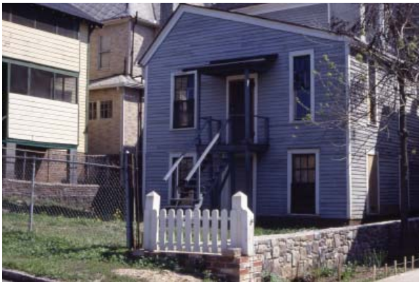
Figure 37. North elevation, oblique view (MALU Archives, Slide 526882, April 1985)
