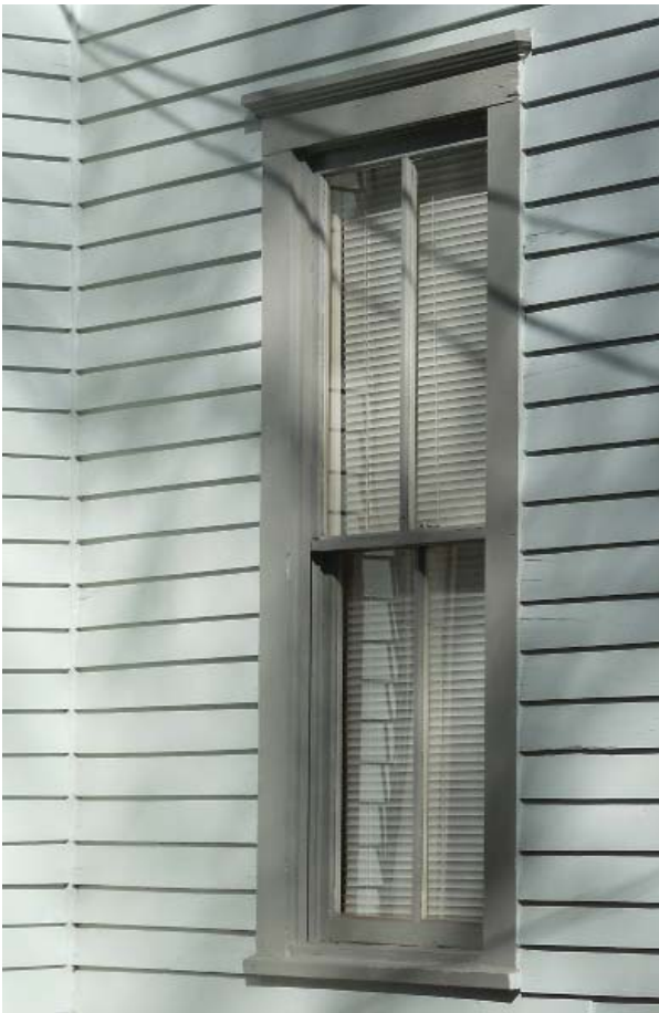
Figure 62. Typical double-hung window.
