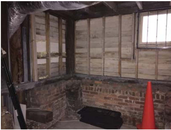
Figure 55. Wall on northeast side of Unfinished Room 004.
