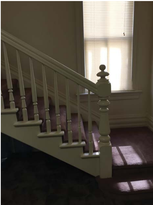
Figure 84. Stair Hall 103 existing stair.
