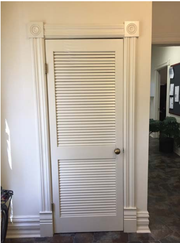
Figure 77. Entry Hall 101 oblique view toward northeast.
