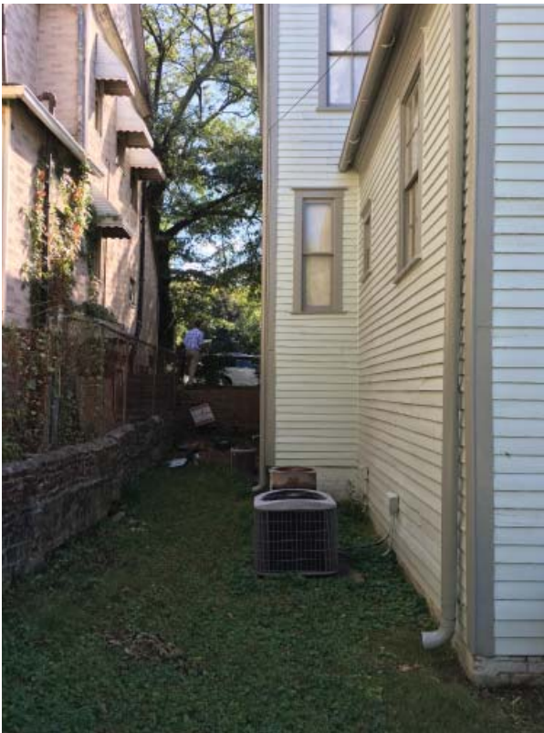
Figure 57. East Side Yard.
