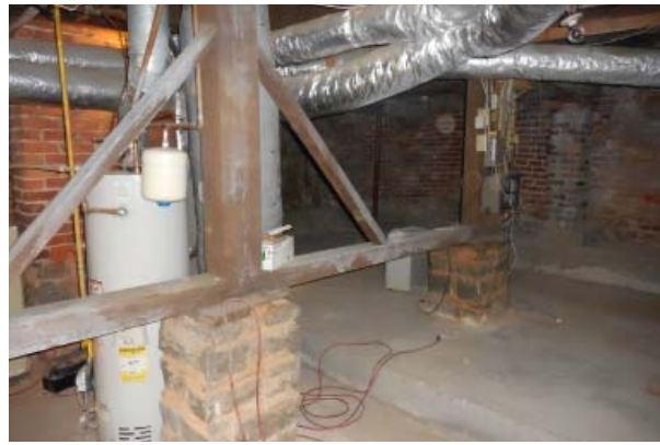
Figure 50. Wood support frame under bearing wall running North-South.
