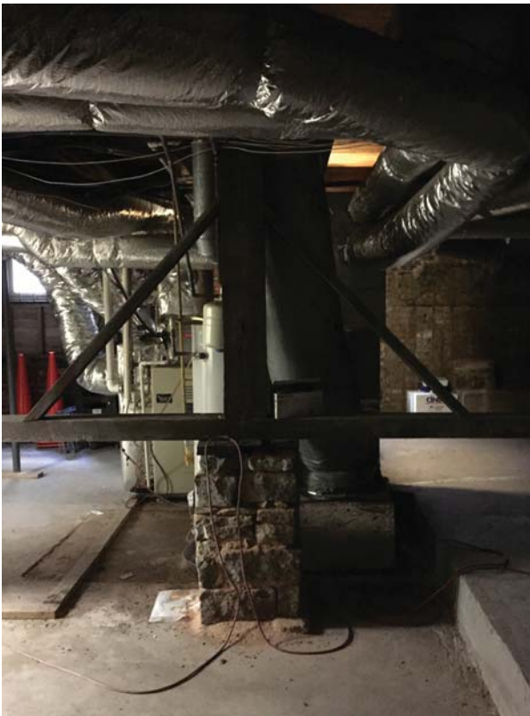
Figure 73. Unfinished Room 004 view toward east.
