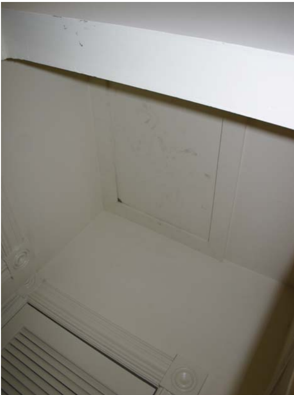
Figure 106. Office 204, attic access panel.
