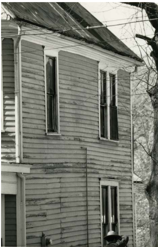
Figure 31. Undated (c. 1985) photo of the east facade of 526 Auburn Avenue prior to exterior improvement project.
