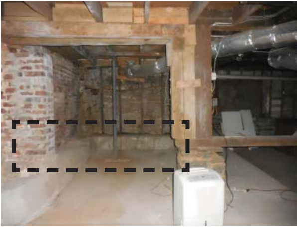
Figure 52. Wood support frame under bearing wall running North-South southern end. Low beam has been removed. Outline of area added for emphasis.
