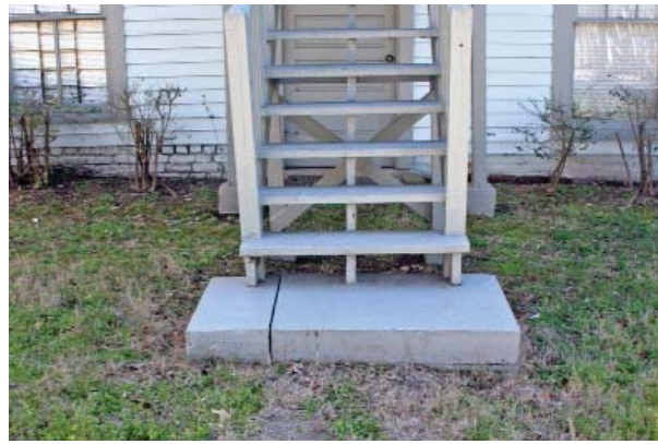
Figure 38. North elevation, rear steps, concrete pad and pavers.
