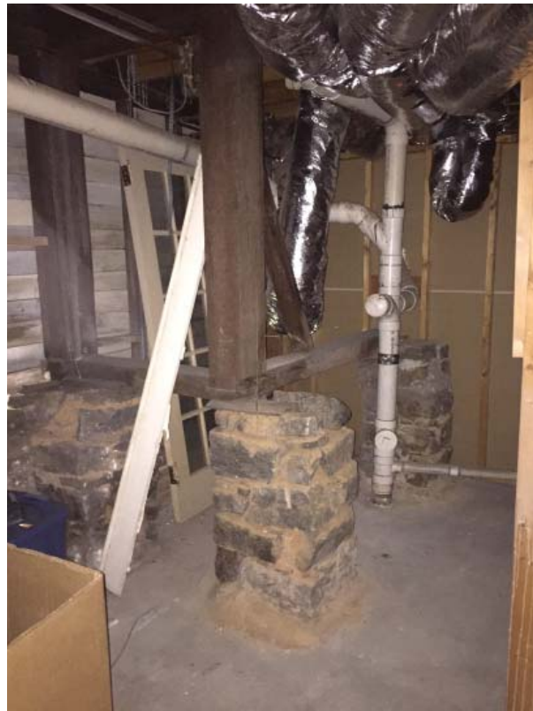
Figure 51. Wood support frame under bearing wall.
