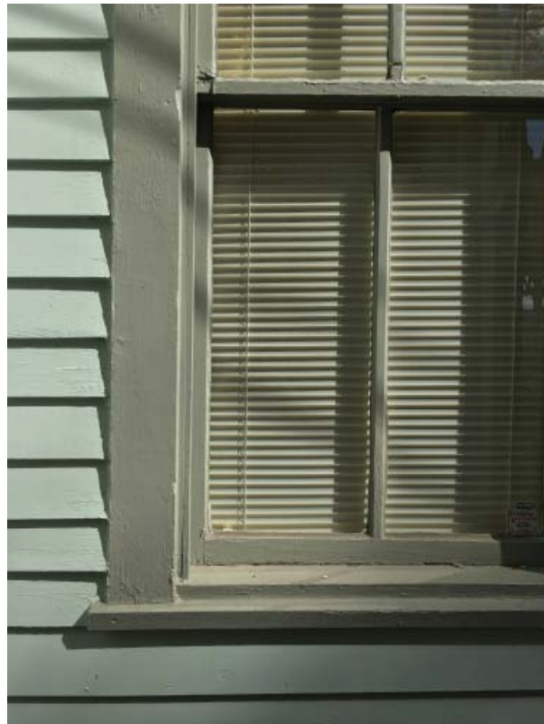
Figure 45. Typical window, exterior view.
