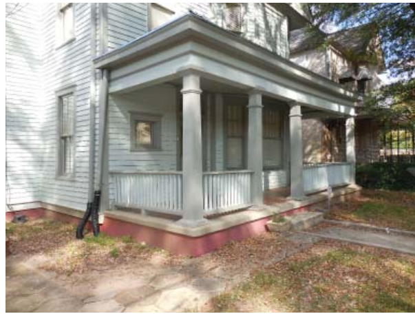
Figure 65. Entry Porch, Oblique View toward east.
