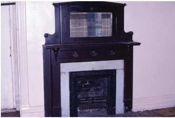
Figure 80. North wall with hearth (MALU Archives, Slide 526-12, April 1985).
