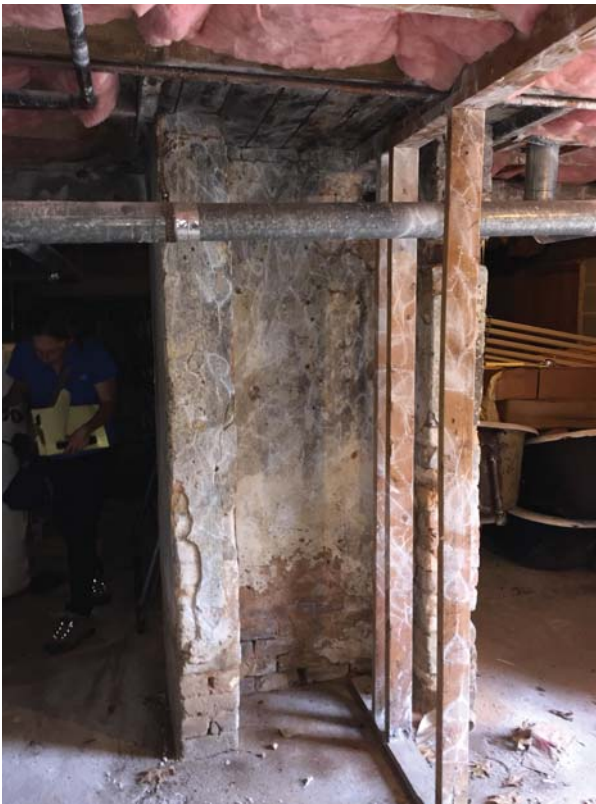
Figure 52. Brick firebox base in Basement 001.
