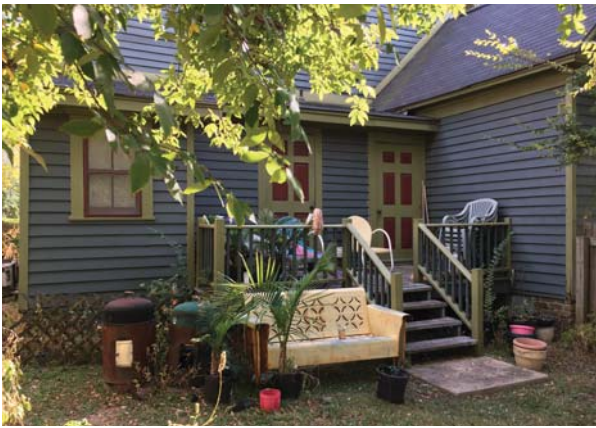
Figure 62. Rear porch, north elevation.
