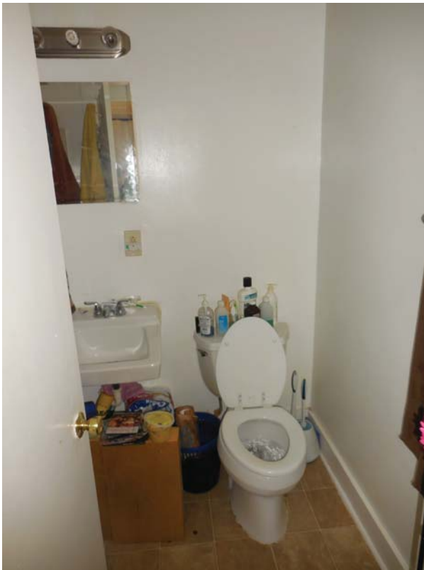
Figure 55. Typical bathroom fixtures.
