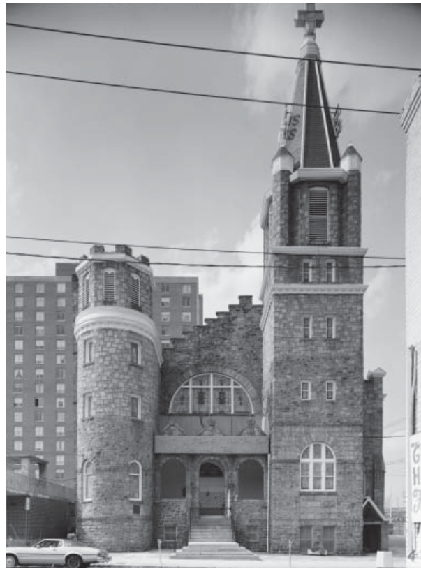
Figure 10. View of the A.M.E. Bethlehem Church, “Big Bethel” (Library of Congress: HABS GA-1170-C-15).
