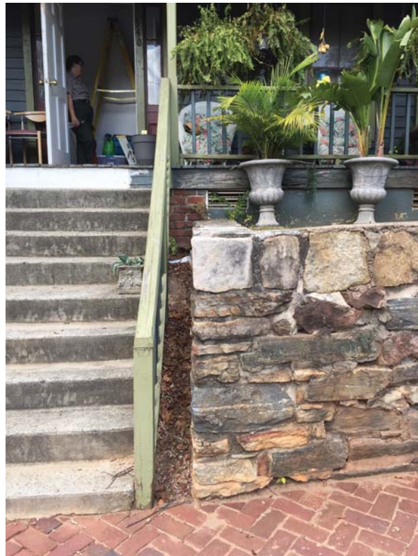
Figure 61. Concrete steps and stone wall, south elevation.
