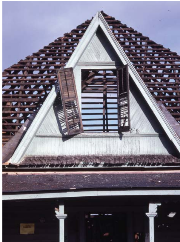
Figure 32. Undated photo of 540 Auburn Avenue during implementation of Self-Help recommendations.
