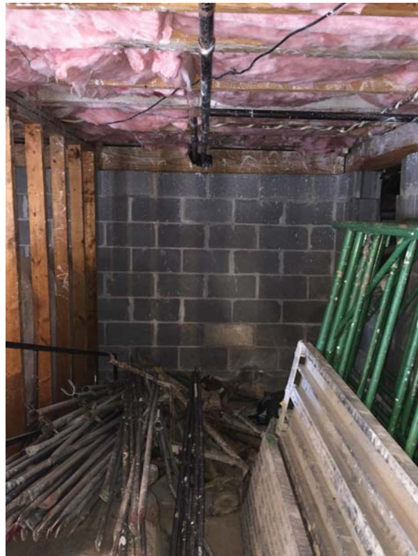
Figure 65. Basement 001 view toward north, crawlspace access to right.
