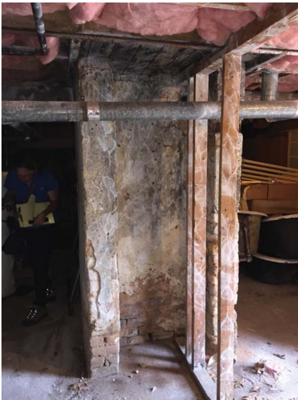
Figure 66. Masonry fireplace structure.
