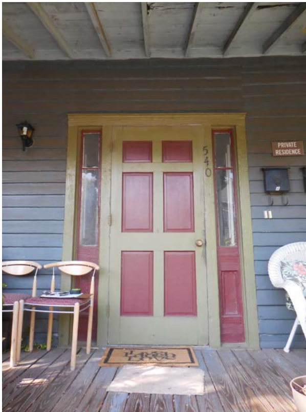
Figure 57. South Elevation, front door.
