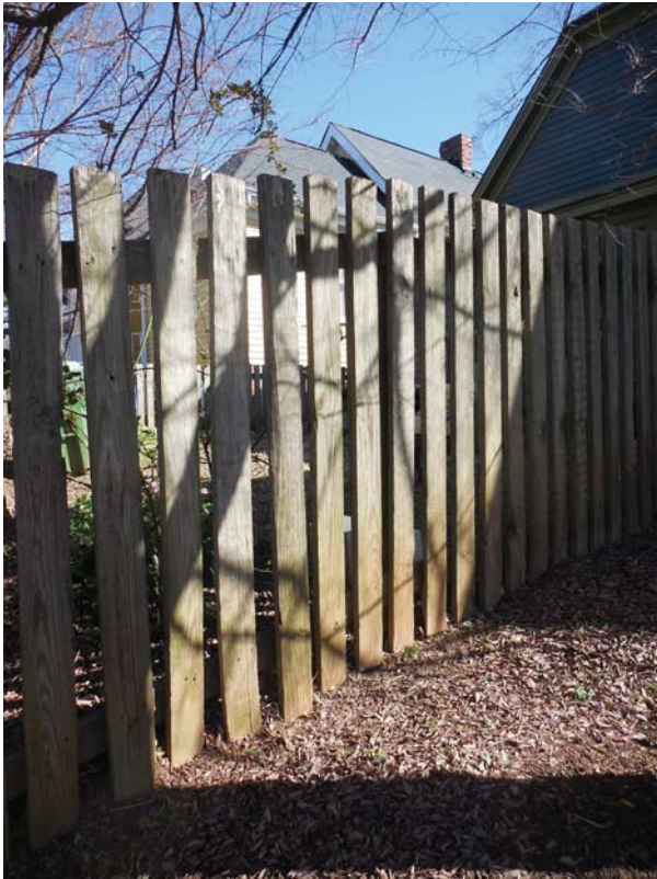
Figure 38. Wood picket fence, west elevation.
