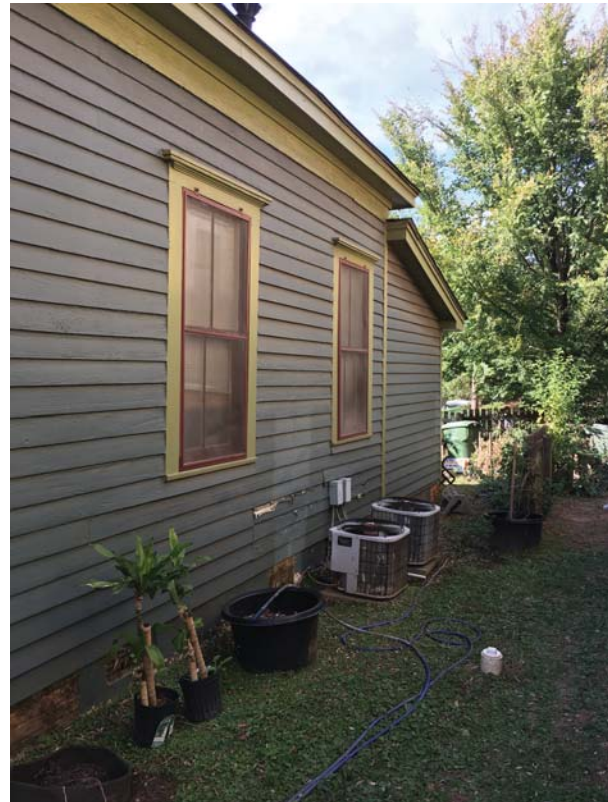
Figure 40. East elevation, oblique view, view toward north.
