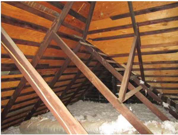
Figure 50. Roof framing in attic, view toward south west corner. Kickers attach to mid height of rafters.
