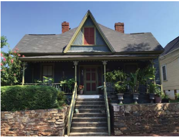
Figure 41. South elevation, porch and gable.
