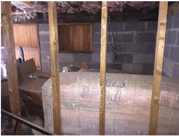
Figure 64. Basement 001 view toward west.
