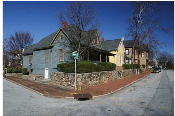
Figure 36. Entire block, including 540, 546, and 550 Auburn Avenue; view toward northeast.
