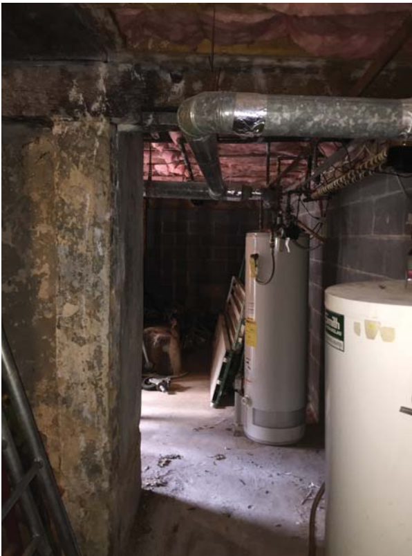
Figure 67. Basement 001, view toward north, masonry fireplace base in foreground.
