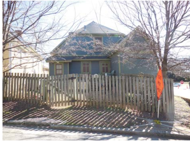
Figure 39. Site, north elevation of house, view toward south.
