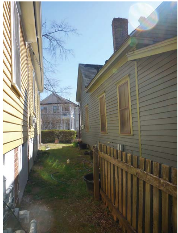
Figure 43. East elevation and yard, oblique view toward southwest.
