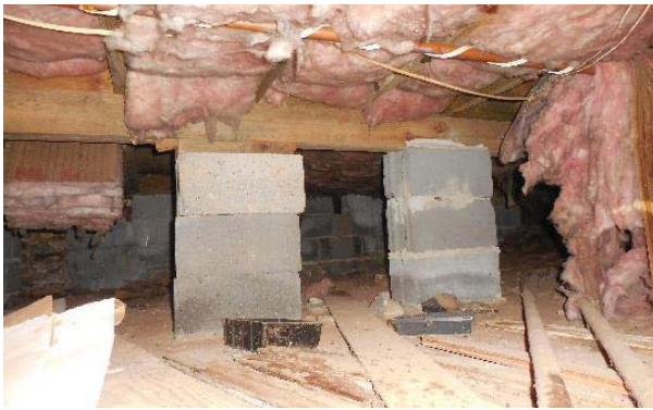
Figure 48. Foundation wall and piers.
