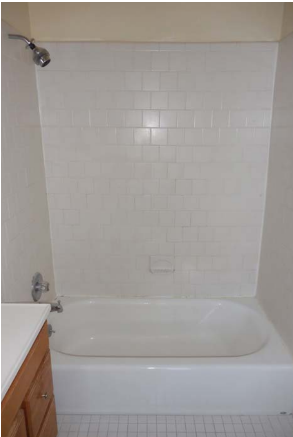
Figure 86. Bath 208, view toward south, bathtub and surround.
