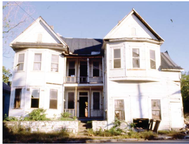
Figure 43. South elevation, prior to Self-Help Project (MALU Archives, Slide 550_19, undated).
