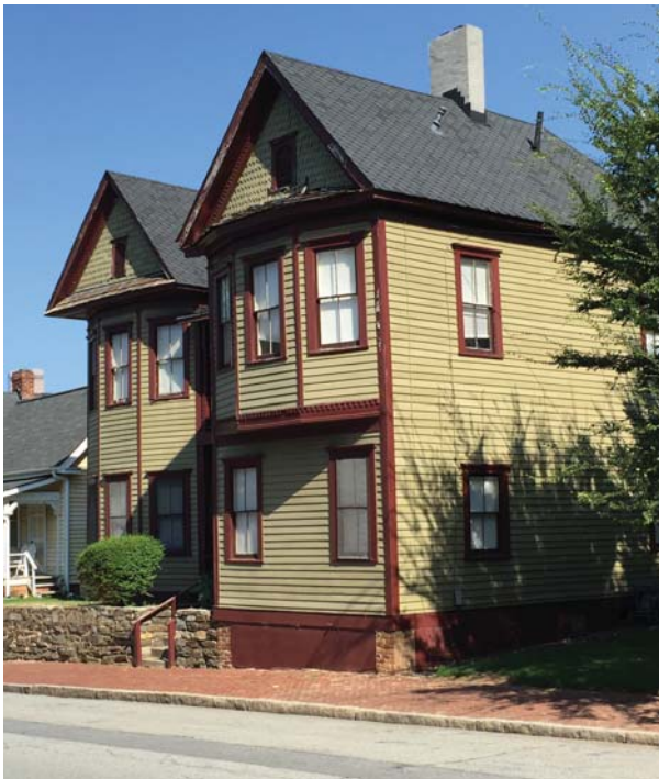
Figure 36. South elevation, oblique view toward southwest.
