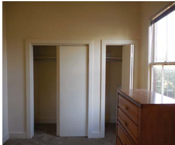
Figure 88. Bedroom 209, view toward south.
