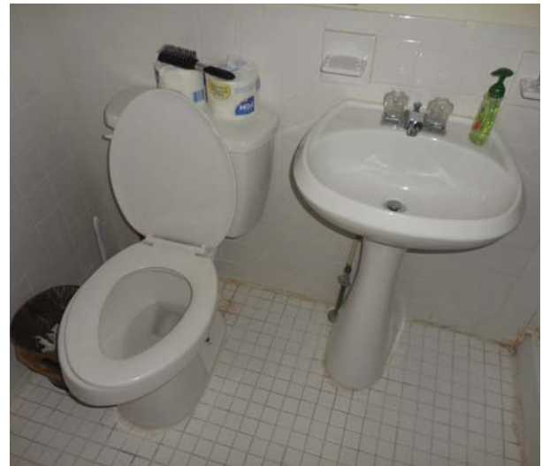
Figure 79. Bath 205, looking east, bathroom fixtures.
