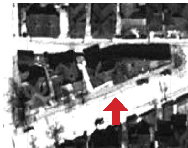
Figure 29. Aerial image of Auburn Avenue Birth Block, 1949 (Georgia State University Special Collections).
