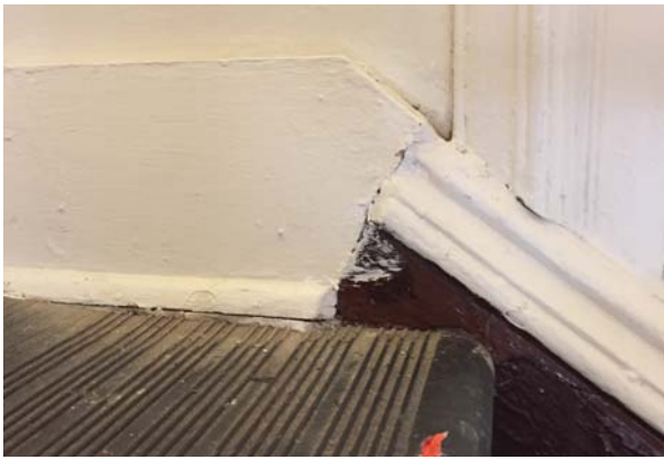
Figure 62. Stair Hall 101/201, top landing of stair, detail.
