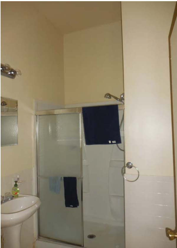
Figure 78. Bath 205, view toward south.
