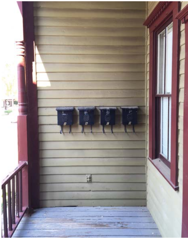
Figure 57. Front porch, first floor, view west.
