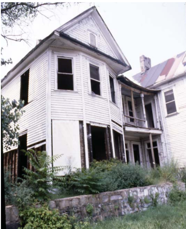
Figure 44. South elevation, prior to Self-Help Project (MALU Archives, Slide 550_27, undated).
