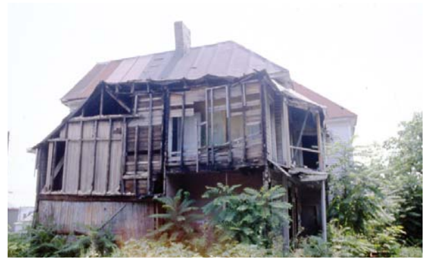
Figure 47. East elevation (MALU Archives, Slide 550_24).
