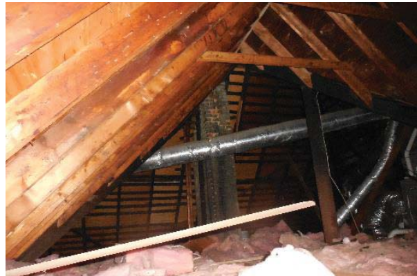
Figure 51. Roof framing in attic.
