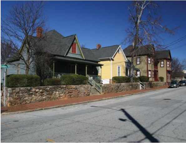
Figure 34. Entire block, including 540, 546, and 550 Auburn Avenue; view toward northeast.
