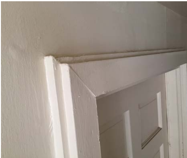
Figure 66. Hall 103, additional door trim, detail.
