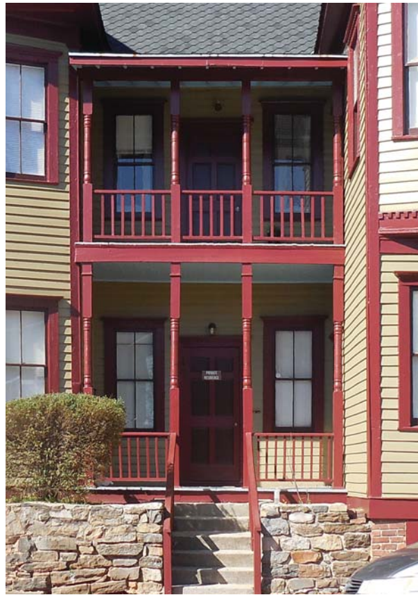
Figure 53. South elevation, front porch.
