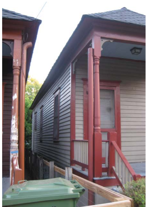
Figure C5. West side yard looking north.
