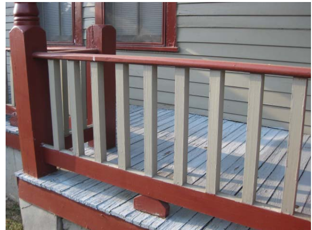
Figure C24. Front porch floorboards and balustrade.
