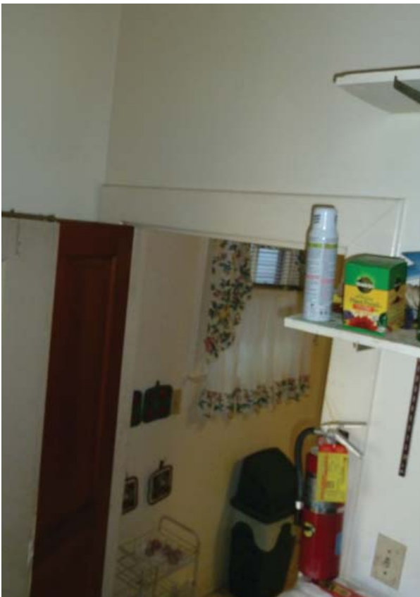
Figure C52. Room 108, southeast oblique.
