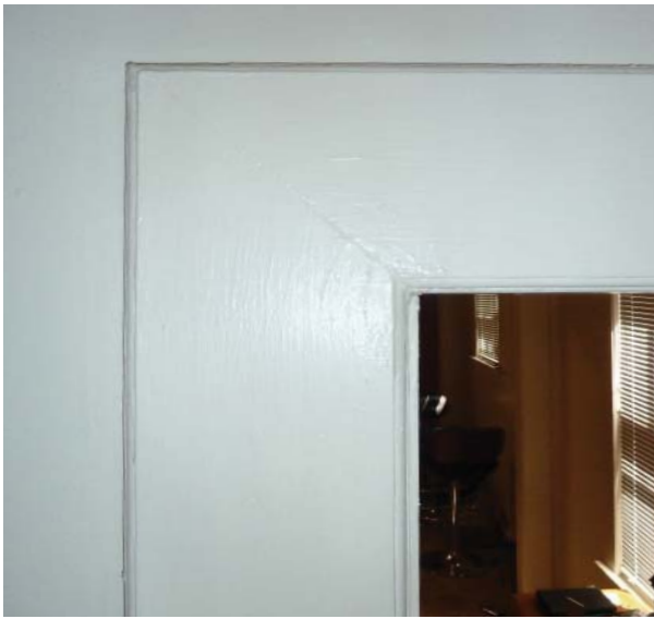
Figure C31. Typical door and window casing.
