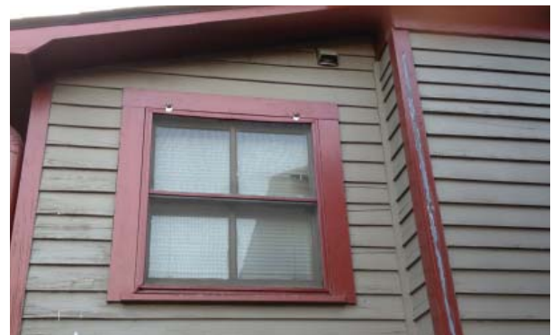
Figure C18. Window type three at the west side of the rear addition.
