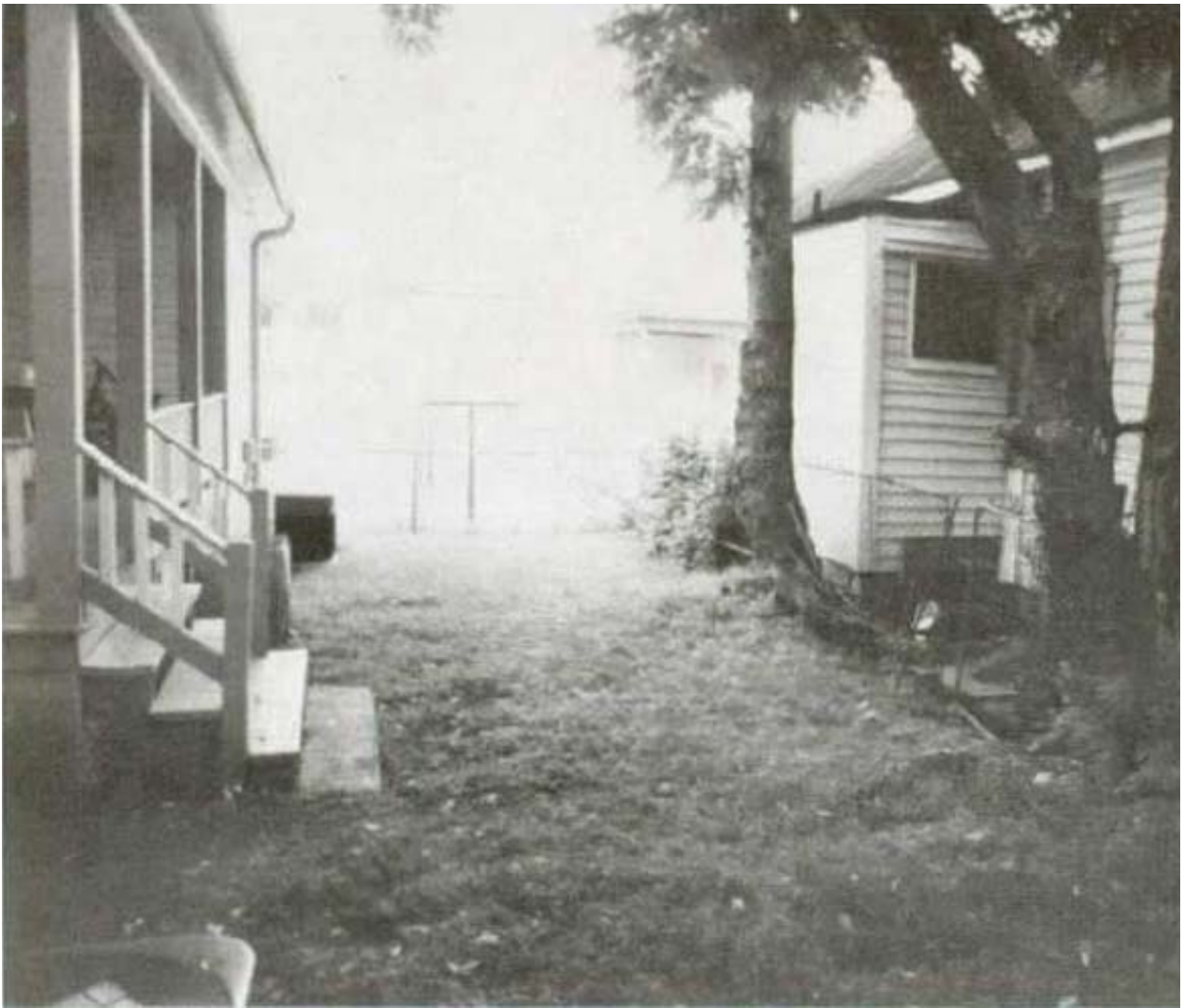
Figure B27. Back yard of the row of the Auburn Avenue double shotguns after the 1991 work (left), showing the new back porch addition and back stair. The distinct yards of the individual residences have been incorporated into one long open strip, no longer dirt but grassed. A clothesline remains in the neighboring yard, and trees and chain link fence identify the property line immediately behind the small shotguns facing Old Wheat Street (right), now demolished. (Lawliss, CLR , p. 42)
