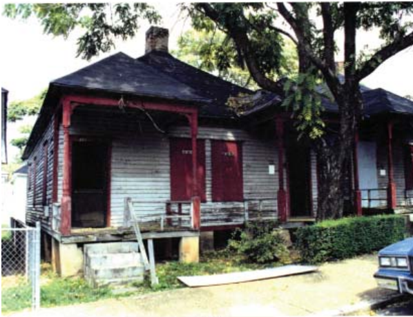
Figure B18. Front and west side of 480-82 Auburn Avenue in 1991 before work. To the right is 484-86. Farther right (east) and not visible is 488-90 Auburn, which was in similar condition. (HSAR)
