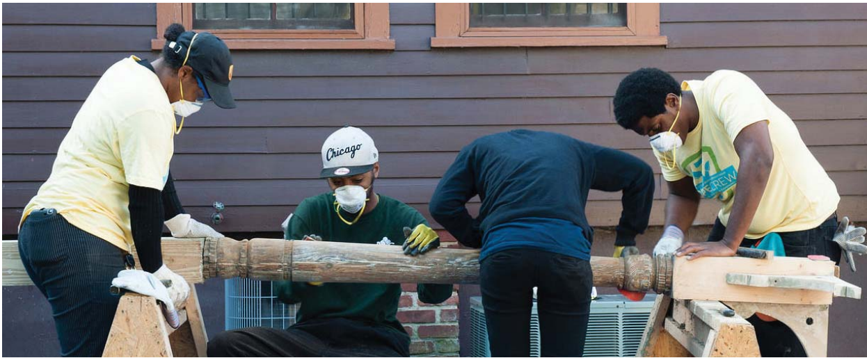
Figure B28. Members of the HOPE Crew sanding a turned porch post of one of the shotgun houses on Auburn Avenue. ("HOPE Crew Restores Historic Shotgun Houses in Atlanta," 6 November 2014, savingplaces.org )
