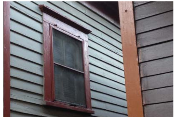
Figure C17. Window type two on the north portion of the east and west side of the main block. Obscured by the screen, this is a two-over-two double sash wood window.
