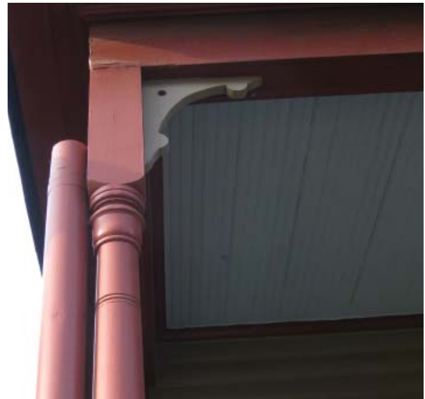
Figure C23. Decorative bracket and crown molding at front porch.
