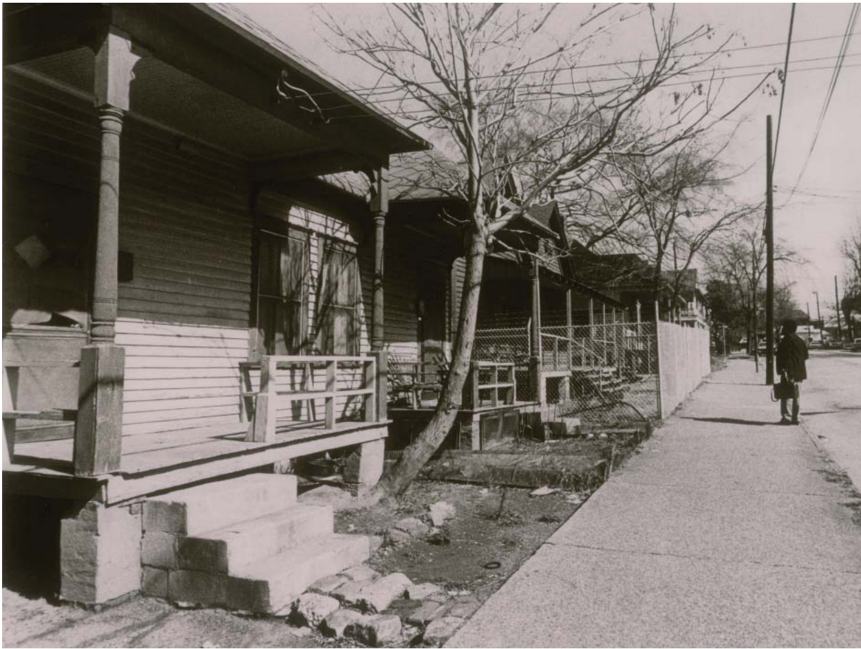
Figure B16. The double shotgun houses in the 1980s, or more likely earlier, showing front yards and separate porches. Undated photograph. (MALU Collection)
