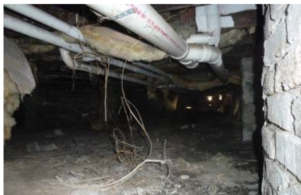
Figure C8. View into crawl space. Note the modern PVC plumbing lines and the modern insulation. Photograph taken at 484 Auburn Avenue, where access was provided.
