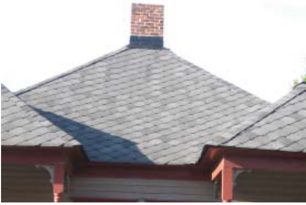
Figure C27. "French Method" composition shingle roof and front chimney.
