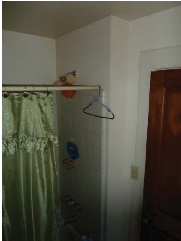
Figure C54. Room 110, southwest oblique.
