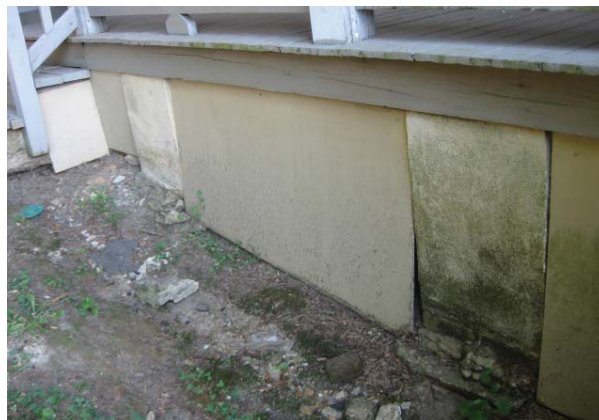
Figure C7. Typical stuccoed masonry foundation pier or rear addition. Photograph taken at 484 Auburn Avenue, where access was provided.
