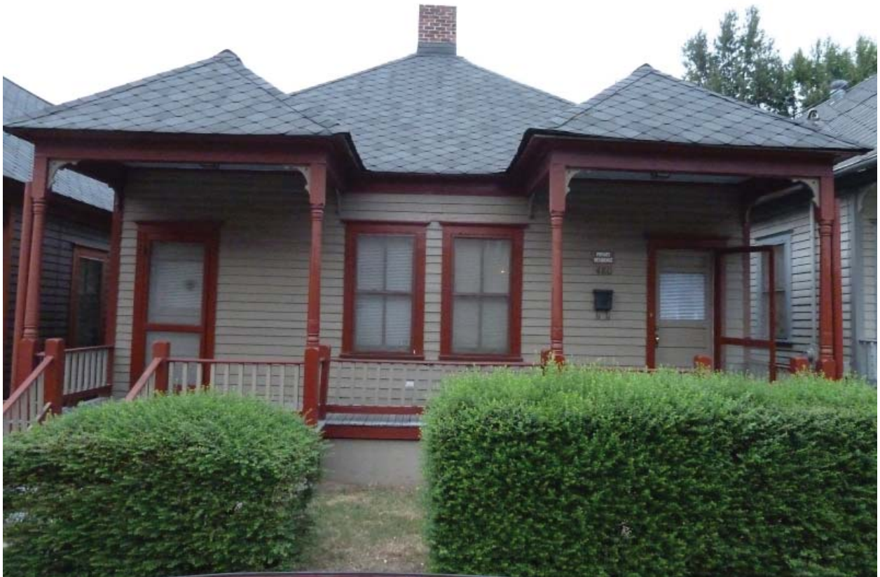
Figure C1. 480 Auburn Avenue viewed from south side of street. Unless otherwise specified, all photos in this section taken by JKOA in 2016.
