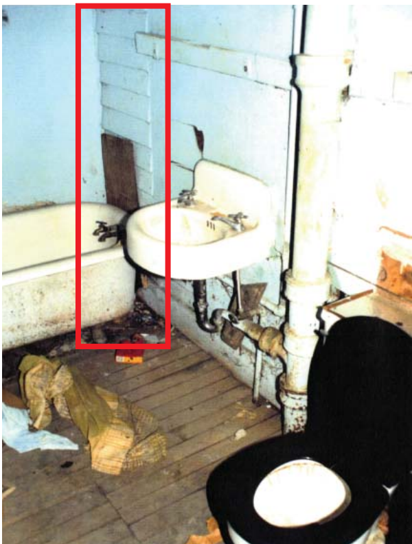
Figure B13. West bathroom of 480 Auburn before 1991 work, showing expansion into back porch when bathtub added. Red border outlines east exterior siding of porch and change in flooring. (HSAR)
