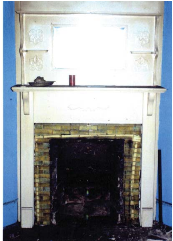
Figure B19. Corner mantelpiece in front room of 484 before work began, showing the mantel and upper shelves in place, firebox with tile surround, board floor, baseboards and plaster walls. (HSAR)
