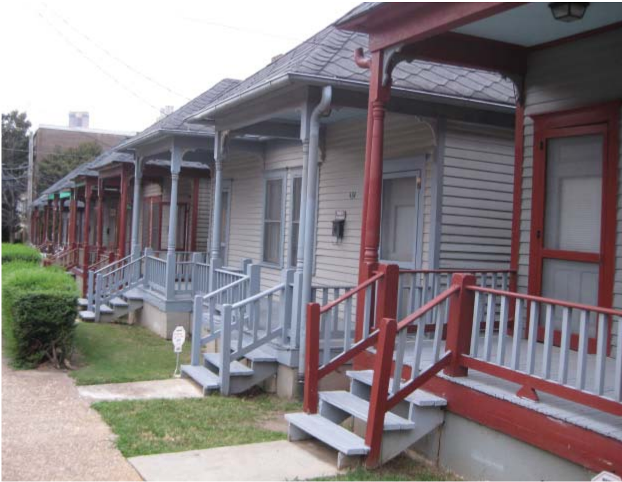
Figure M4. The row of 1905 double shotguns facing Auburn Avenue, each with its two hipped-roof entrance porches, now connected. The third house from the right, with red trim, is 480 Auburn. (JKOA 2016)
