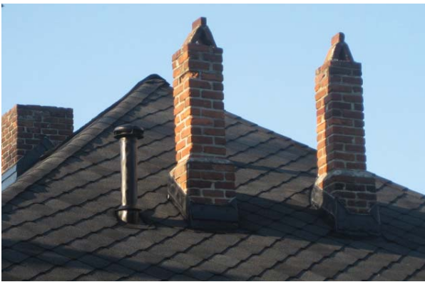
Figure C29. Paired rear brick chimneys with corbelled integrated cap.
