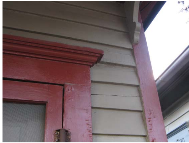
Figure C13. Weatherboard siding and plank cornerboards.
