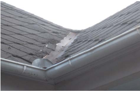
Figure C28. Typical valley flashing of roof. Photograph taken at 484 Auburn Ave.
