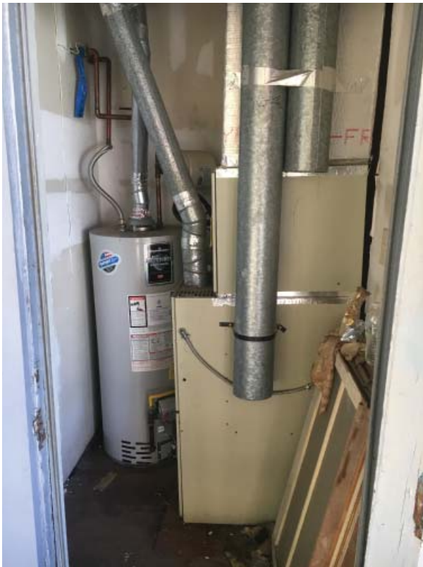
Figure C53. Room 109, looking south. Photograph taken at 484 Auburn Ave.
