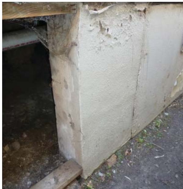
Figure C6. Typical stuccoed masonry foundation pier of main block and cement board infill wall. Photograph taken at 484 Auburn Avenue, where access was provided.
