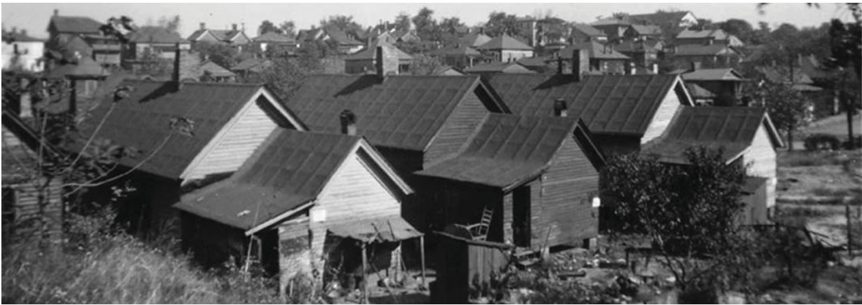
Figure B8. Roll roofing covers houses in this ca. 1940 photograph. Photographs taken during the period of significance of the Birth-Home Block show a preponderance of roll roofing in African-American neighborhoods, and the 1995 CLR reports roll roofing still evident on many Auburn buildings. (Atlanta History Center)
