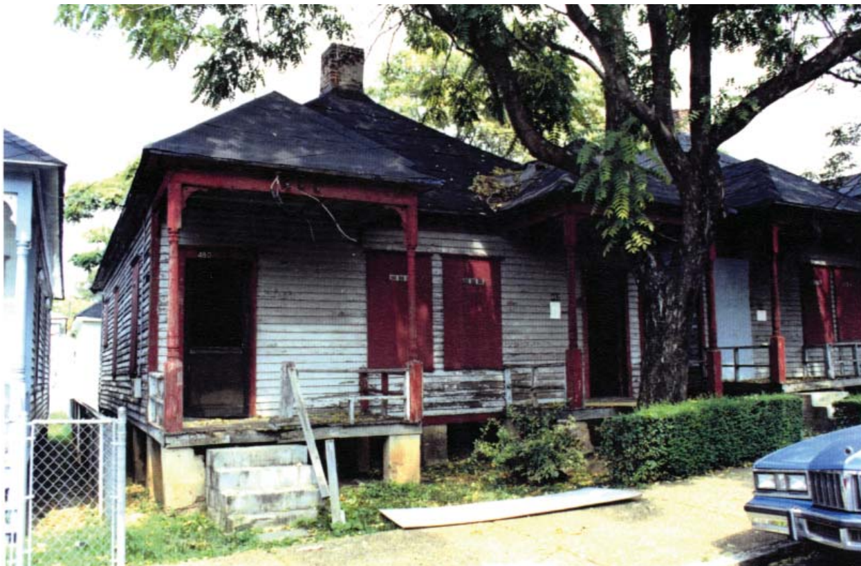
Figure M2. Double shotguns at 480 (left) and 484 Auburn Avenue in 1991. Each entrance has its own hipped-roof porch, and all roofs are sheathed with roll roofing. Note central chimney that served two fireplaces in each residence. (MALU collection of 2005-2010 photographs)
