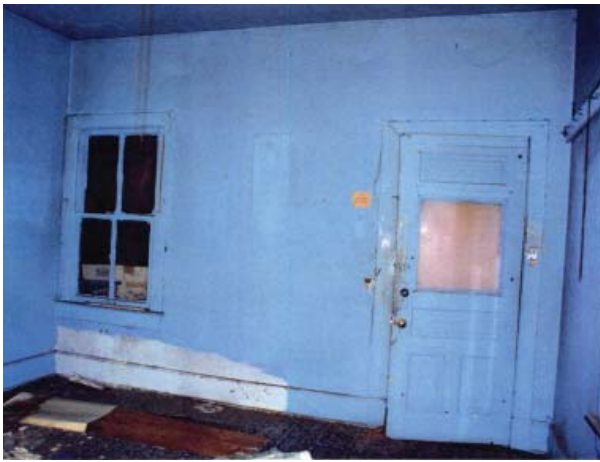
Figure B21. West front room of 484 Auburn Avenue, looking south towards the front door and two-over-two front window. (HSAR)
