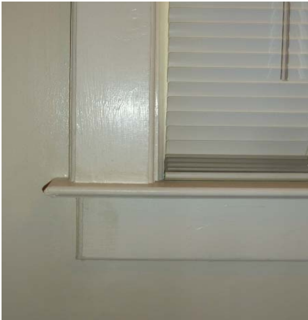
Figure C32. Typical windowsill and apron.
